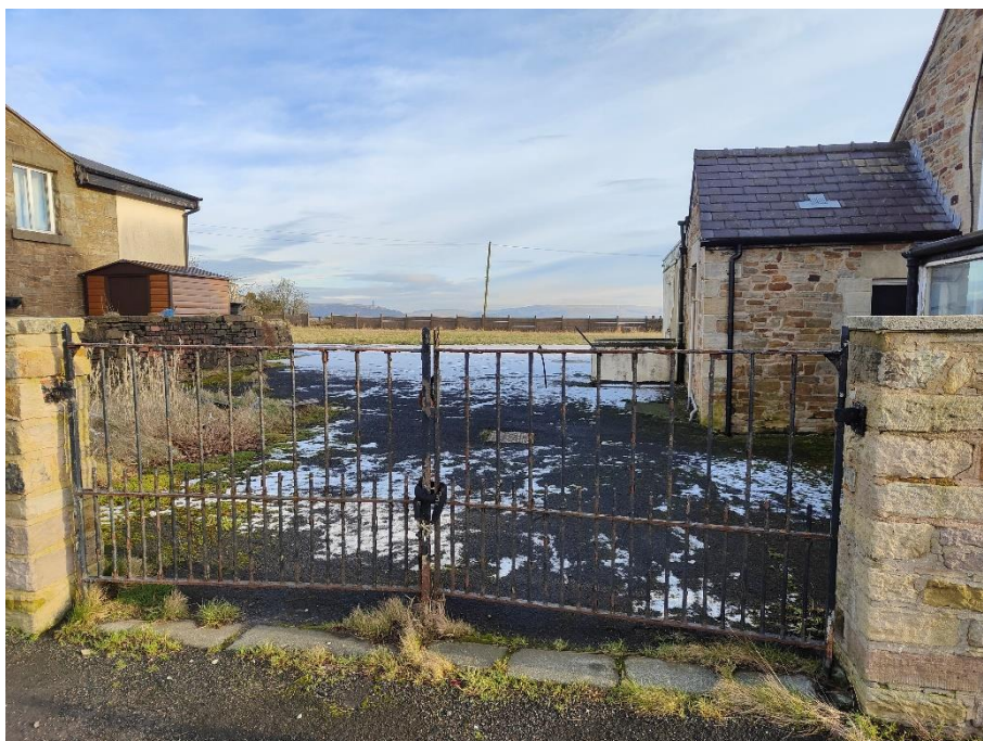
Photograph 2 - Photograph showing access gate from Watling Street, facing northeast
