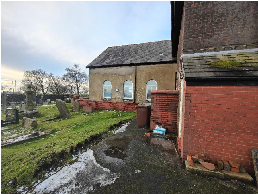
Photograph 5 - Photograph showing the Chapel and graveyard, facing south
