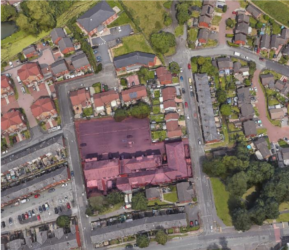
Figure 1.0 – Pre Demolition Site
