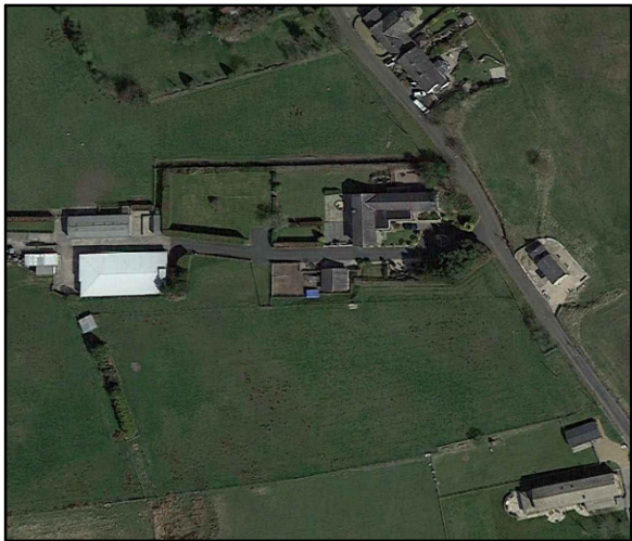
NORTH SOUTH AERIAL VIEW
