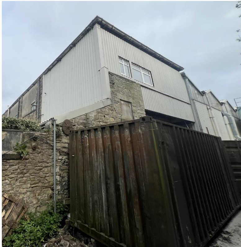
Figure 10 | Existing storage porta cabin
