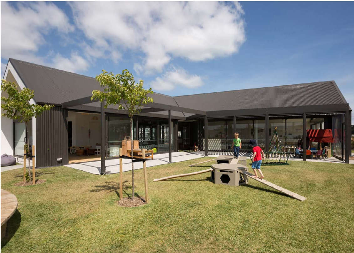
Hobsonville Point ELC, New Zealand
