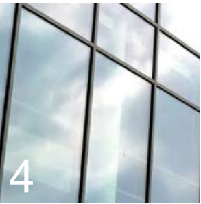
Dark grey parapet capping and window frames
