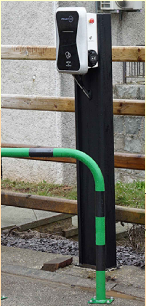
TYPICAL POST MOUNTED EV CHARGING POINT EXAMPLE
