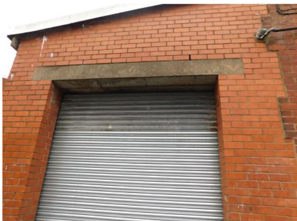
PHOTO 13 Southern View of Garage Door.
