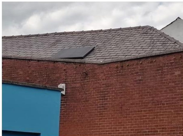
PHOTO 6 View of Southern Roof.
