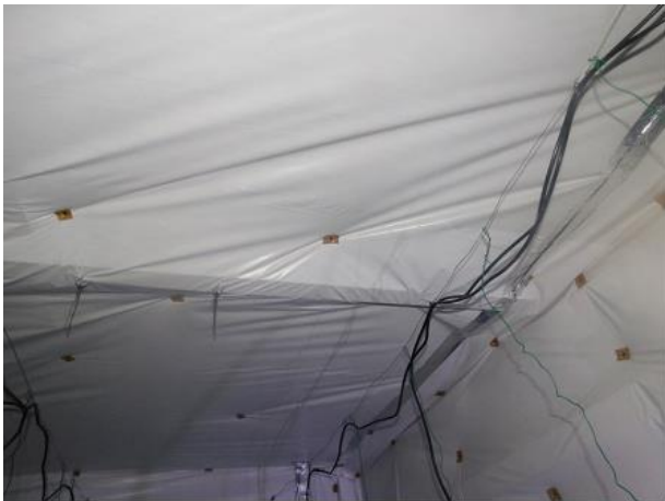
PHOTO 25 Underside of Northern Cellar Roof.
