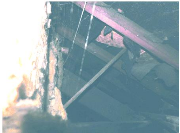
PHOTO 30 Underside of Southern Roof.
