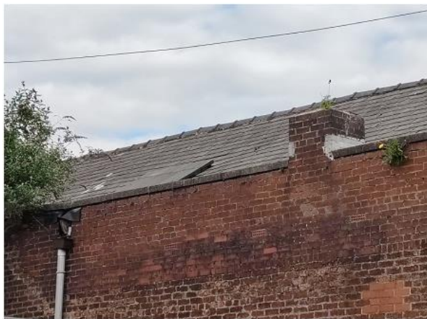
PHOTO 23 View of Northern Roof.
