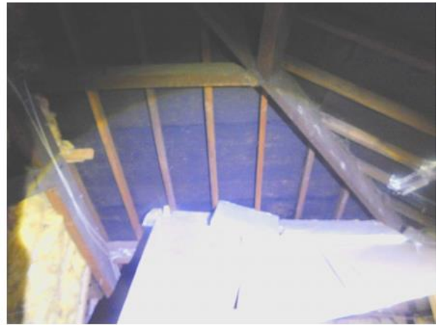
PHOTO 28 Underside of Northern Roof.
