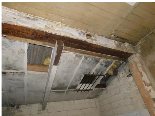
PHOTO 19 Underside of Garage Roof.
