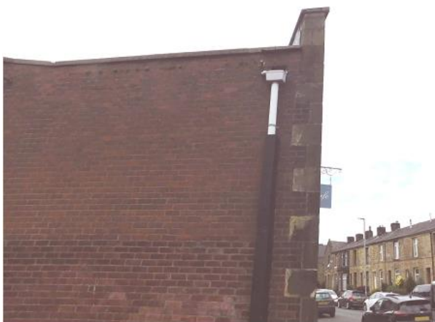
PHOTO 5 South-eastern View of Eastern Parapet Wall.
