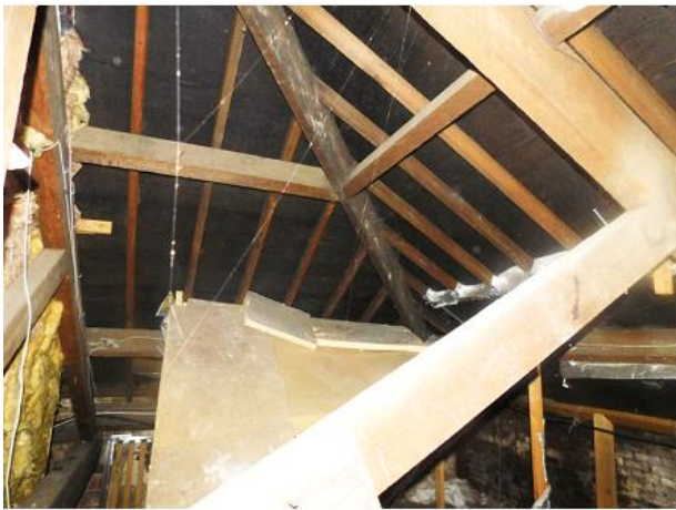
PHOTO 27 Underside of North-eastern Roof.
