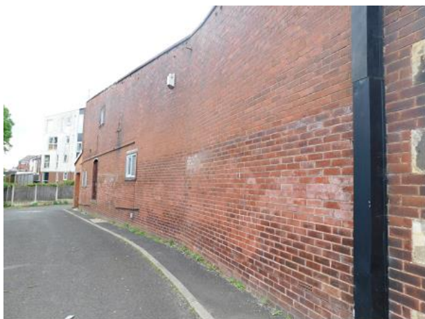
PHOTO 7 Eastern View Along Southern Elevation.
