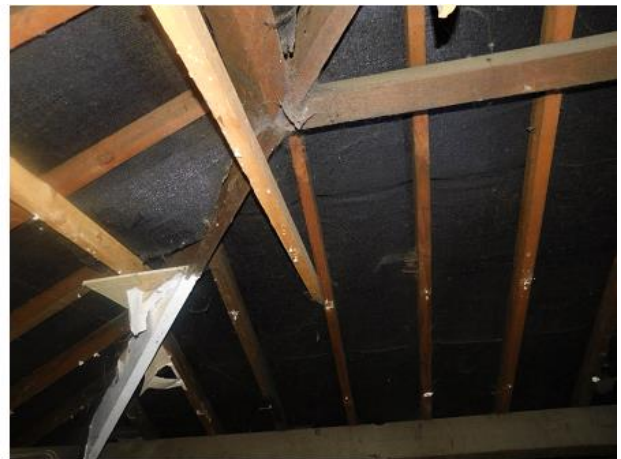
PHOTO 26 Underside of South-eastern Roof.
