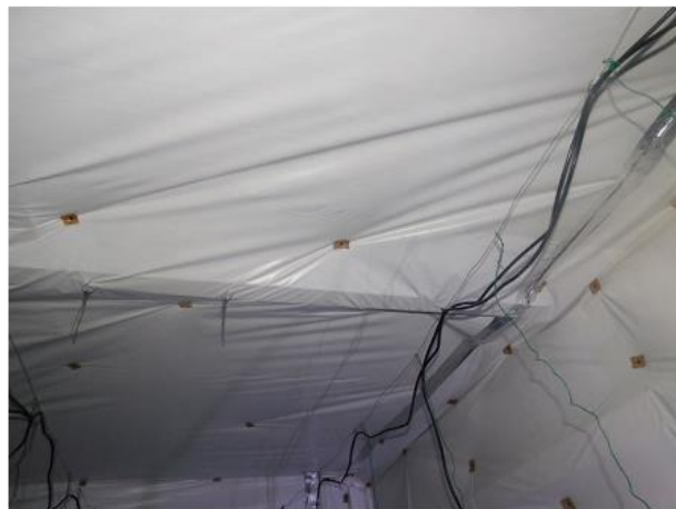
PHOTO 24 Underside of Eastern Cellar Roof.
