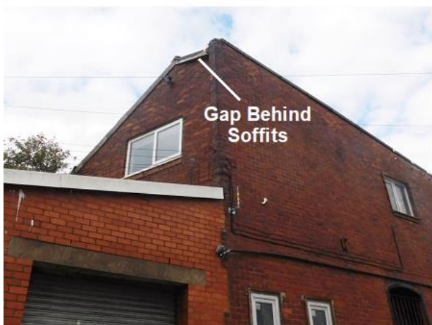
PHOTO 11 Upper South-western Corner.
