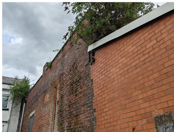
PHOTO 18 Upper Northern Elevation of Garage.
