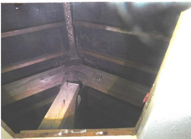
PHOTO 29 Underside of Central Roof.
