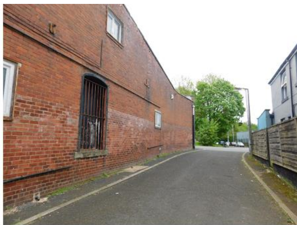
PHOTO 8 Western View Along Southern Elevation.
