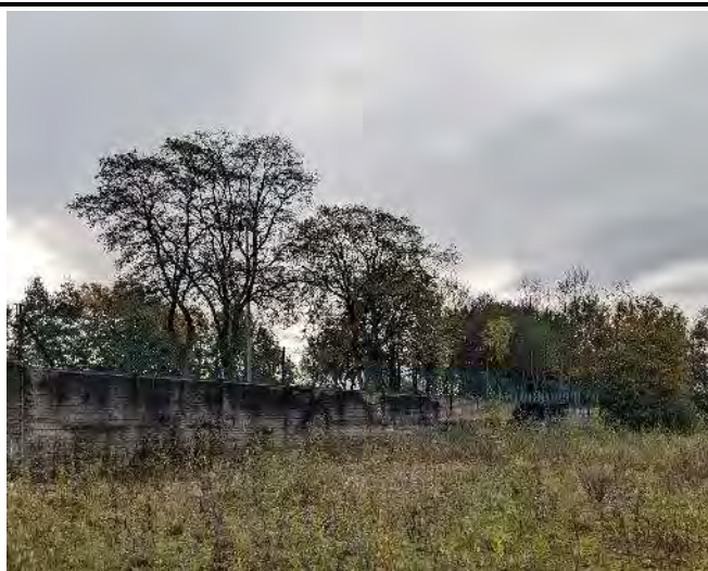
Figure 3 – The retaining wall along the eastern site boundary, looking south-east.
