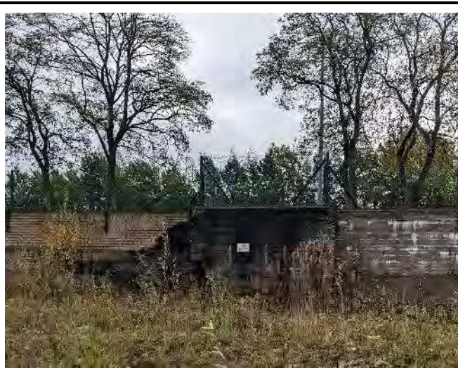
Figure 4 – The eastern retaining wall, looking east.
