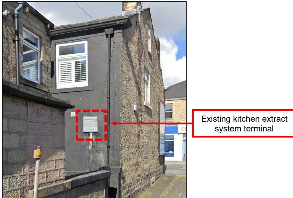
Figure 1.2: Existing Kitchen Extract Location
