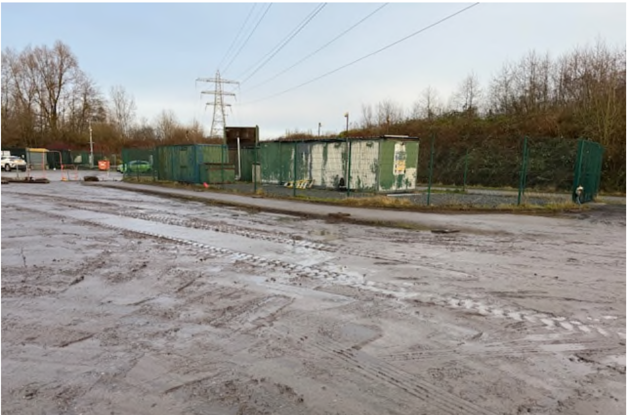
Photograph No 4 - Temporary Buildings on Eastern Part of the Site
