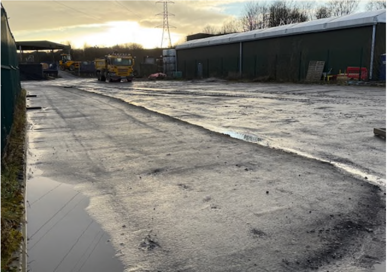
Photograph No 3 - View Across the Site from the North-East Corner
