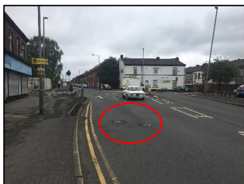
Service covers within new access junction turning area, with localised carriageway deterioration
