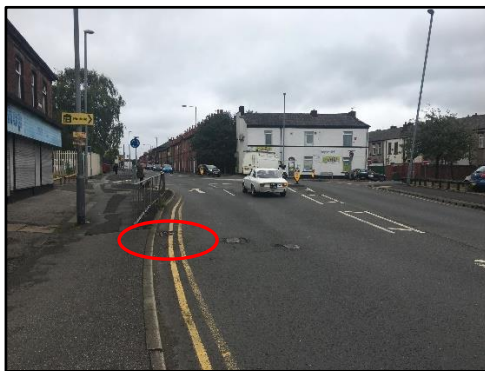
Site visit observed evidence of a blocked gulley
