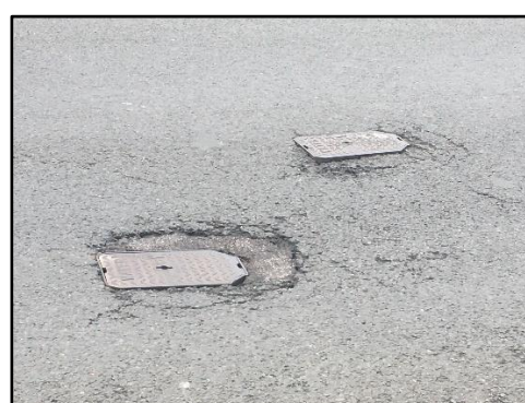
Service covers within new access junction turning area, with localised carriageway deterioration
