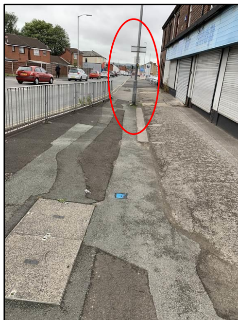
Lamp column in centre of footway
