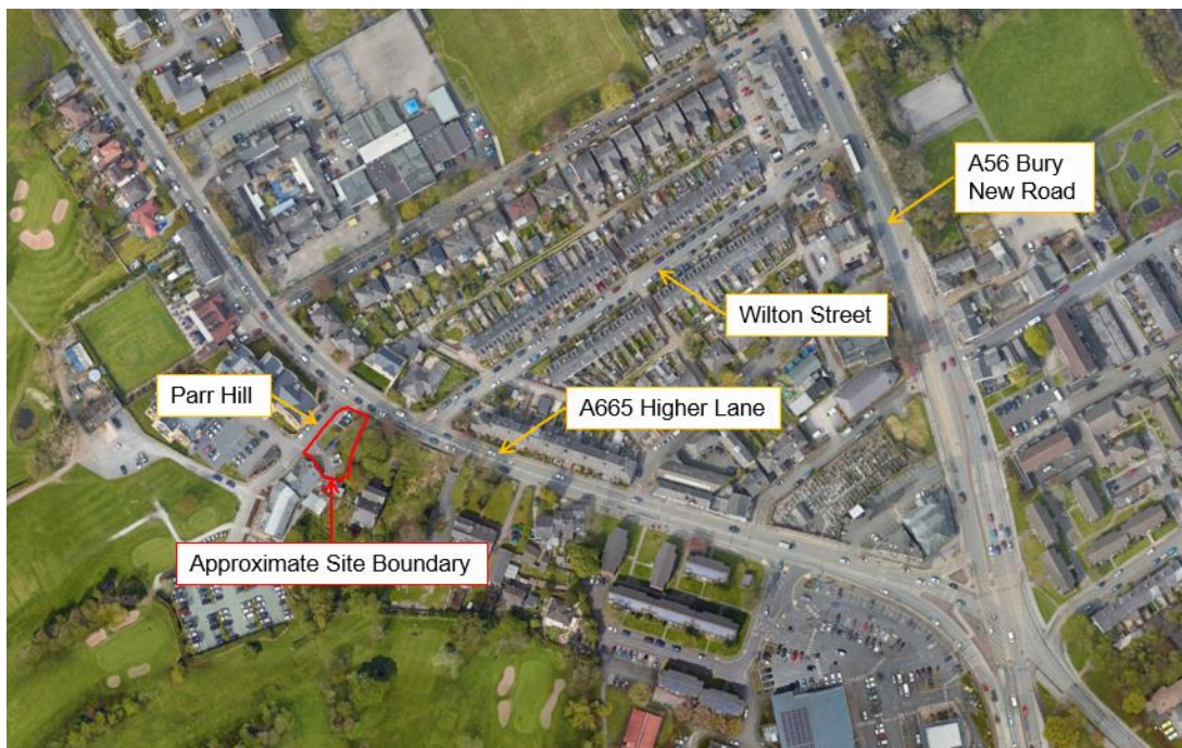
Image 2.1 – Site Location (Local Context)
