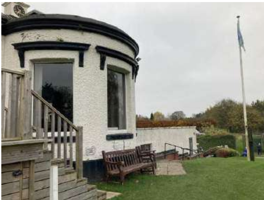
Photograph 4 View south-east towards the western elevation of the existing clubhouse in Site A.
