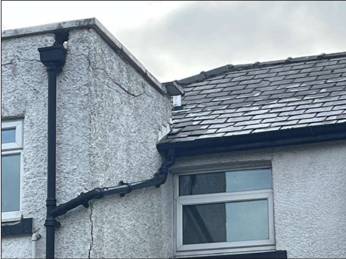
Plate 5 – Example of occasional lifted slates on roof hips
