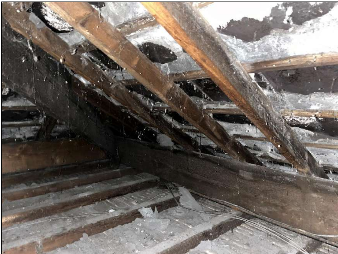
Plate 22 – Internal character of clubhouse loft space
