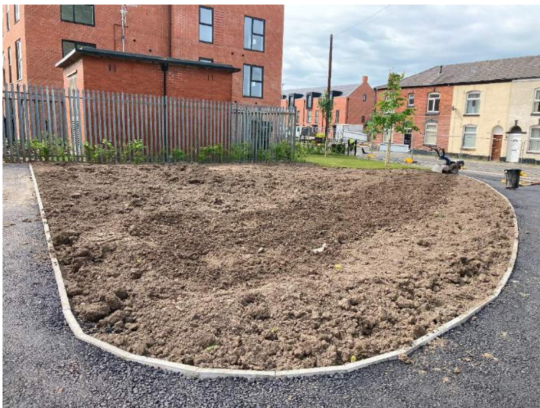
Plate 5 – Area of landscaping in the north of site and area of HP05.
