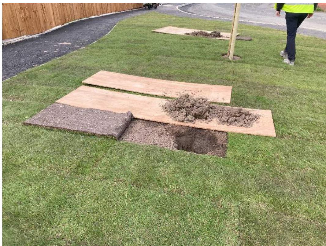
Plate 26 – HP07 GL to 0.30mbgl and arisings, with 0.15m of topsoil.
