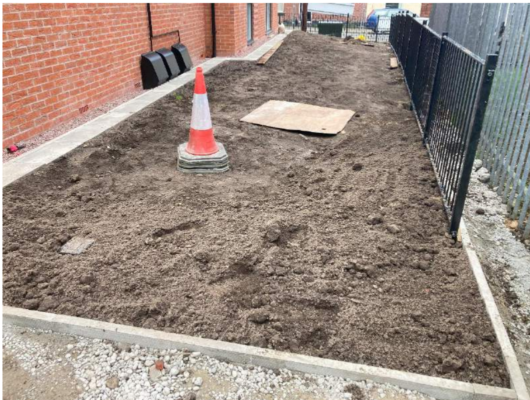
Plate 4 – Landscaping to the north of flats building and area of HP01, looking west.
