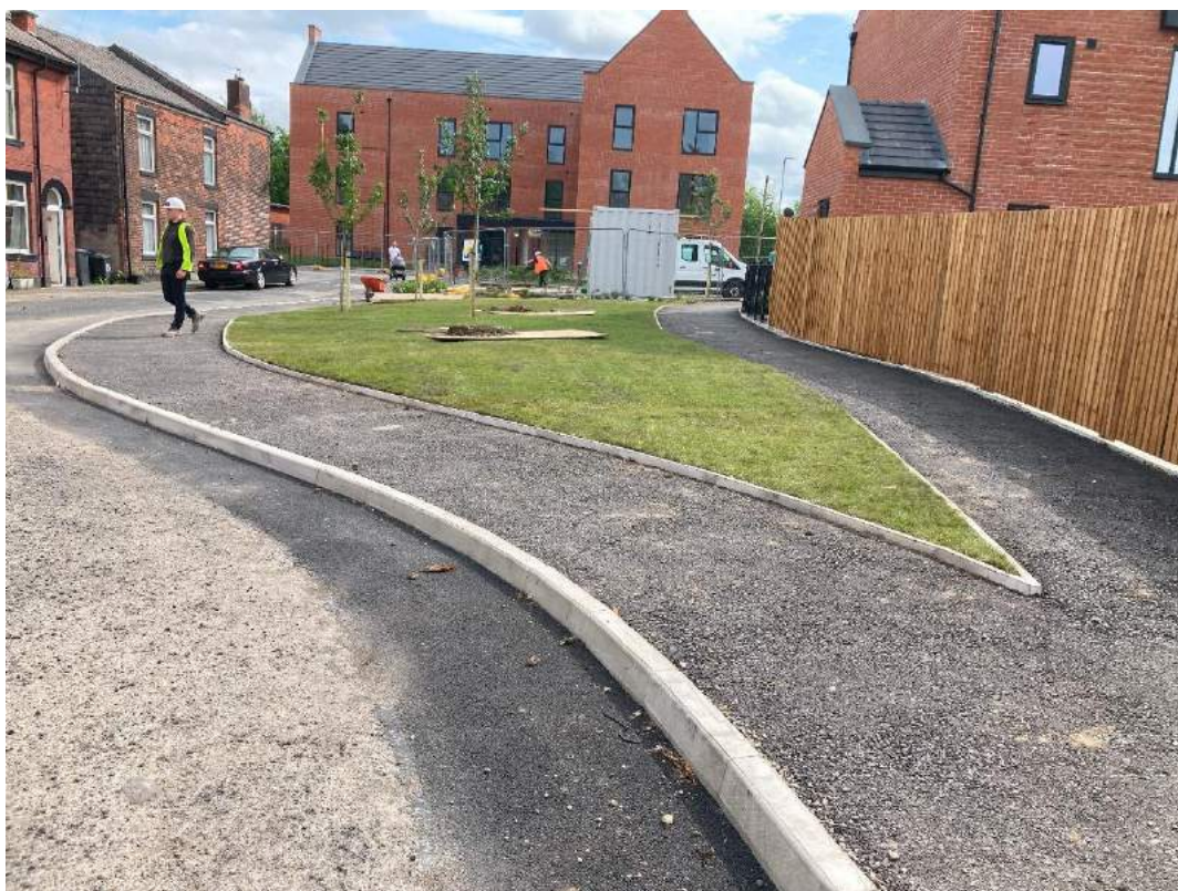
Plate 7 – Area of landscaping within the west of site and area of HP07 and HP08.
