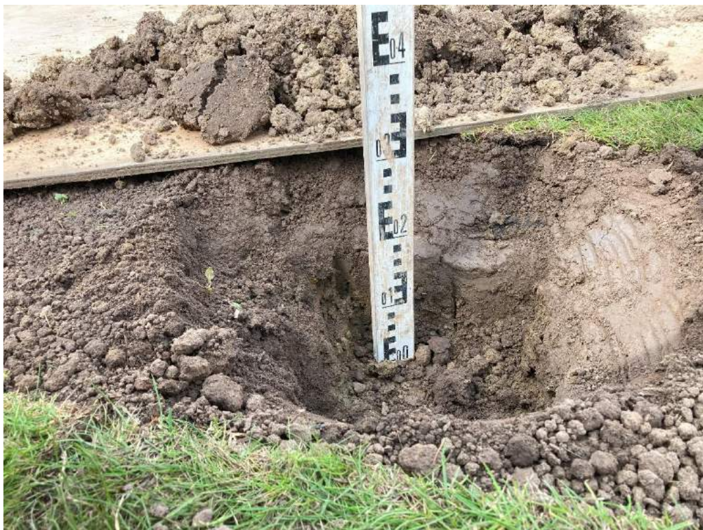
Plate 30 – HP08 GL to 0.3m bgl with 0.15m of topsoil.
