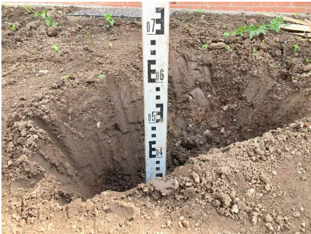
Plate 12 – HP02 GL to 0.6m bgl with 0.15m of topsoil.
