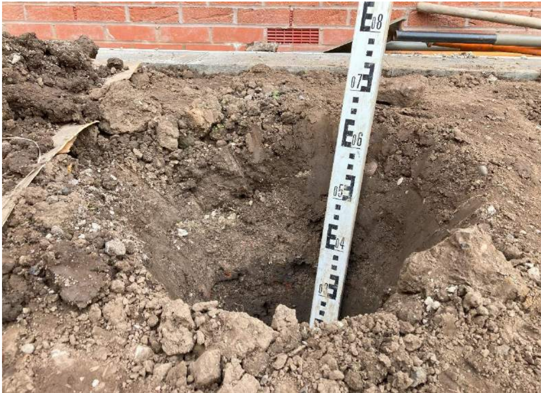
Plate 15 – HP03 GL to 0.6m bgl with 0.15m of topsoil.
