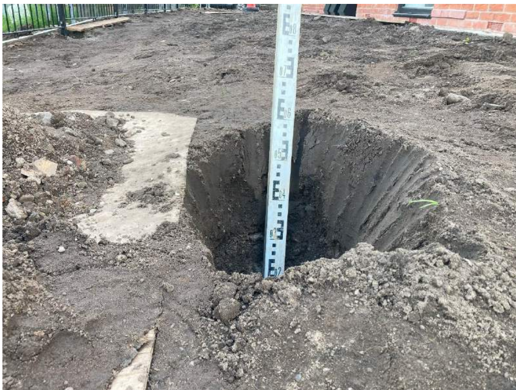
Plate 9 – HP01 GL to 0.6m bgl with 0.2m of topsoil.
