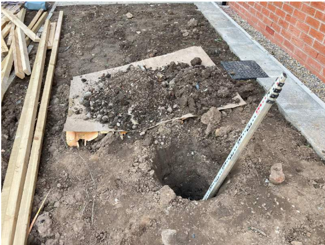
Plate 14 – HP03 GL to 0.60mbgl and arisings, with 0.15m of topsoil.
