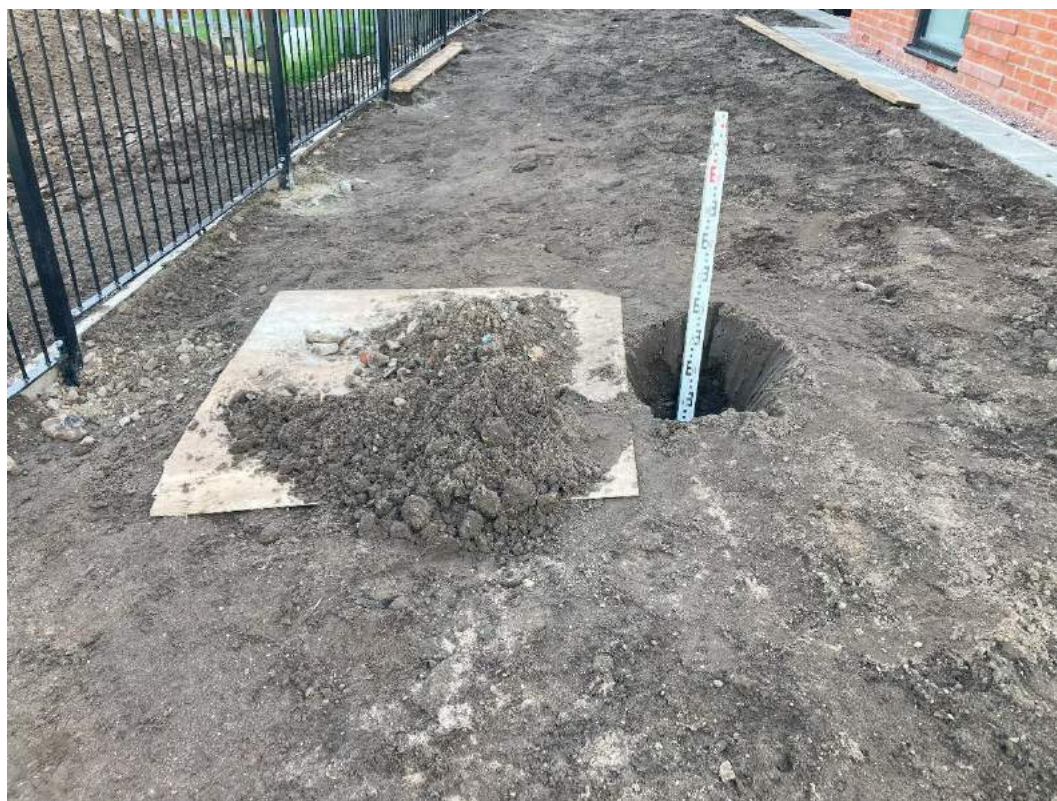
Plate 8 – HP01 GL to 0.60mbgl and arisings, with 0.2m of topsoil.
