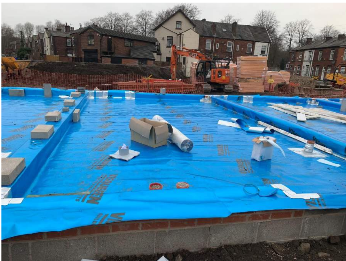
PLATE 3: Plot 5 with Full Visqueen Barrier Coverage
