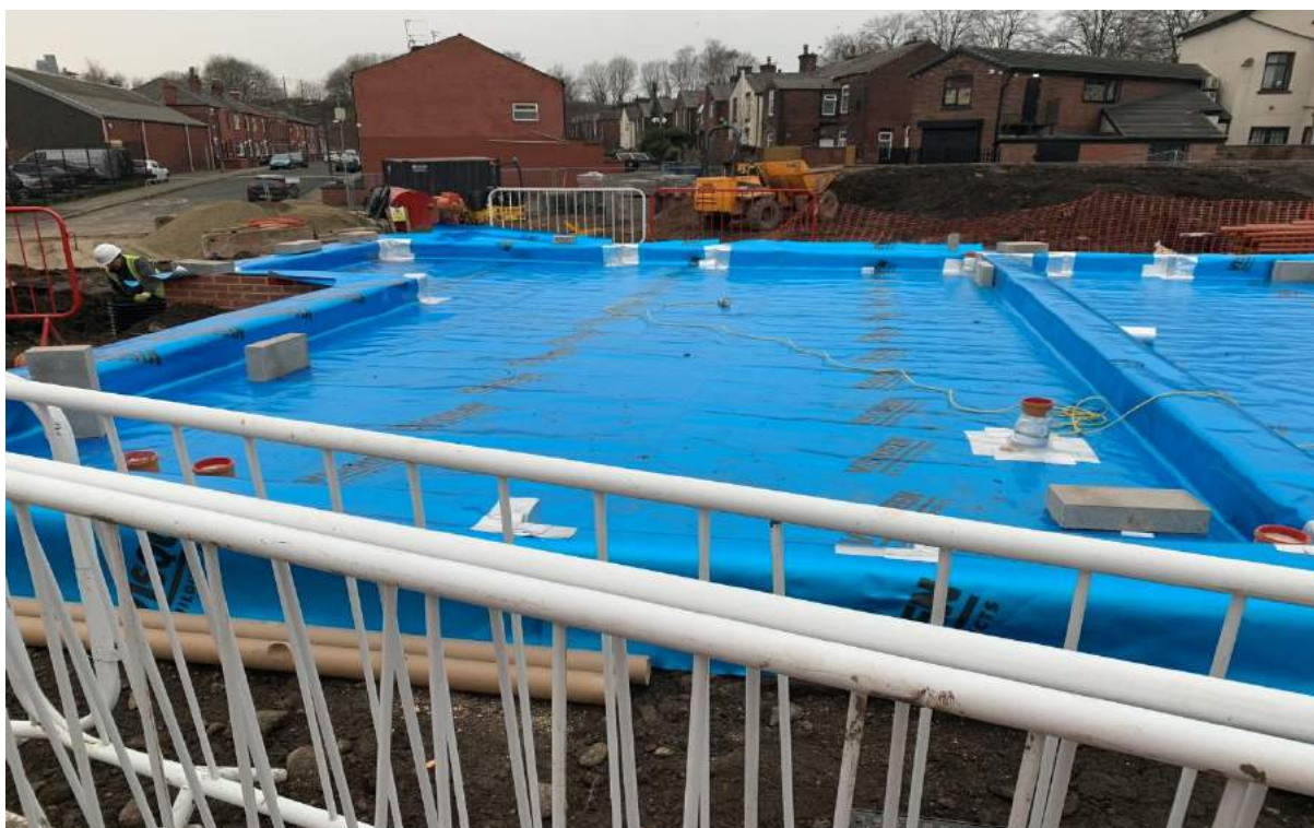
PLATE 5: Plot 7 with Full Visqueen Barrier Coverage
