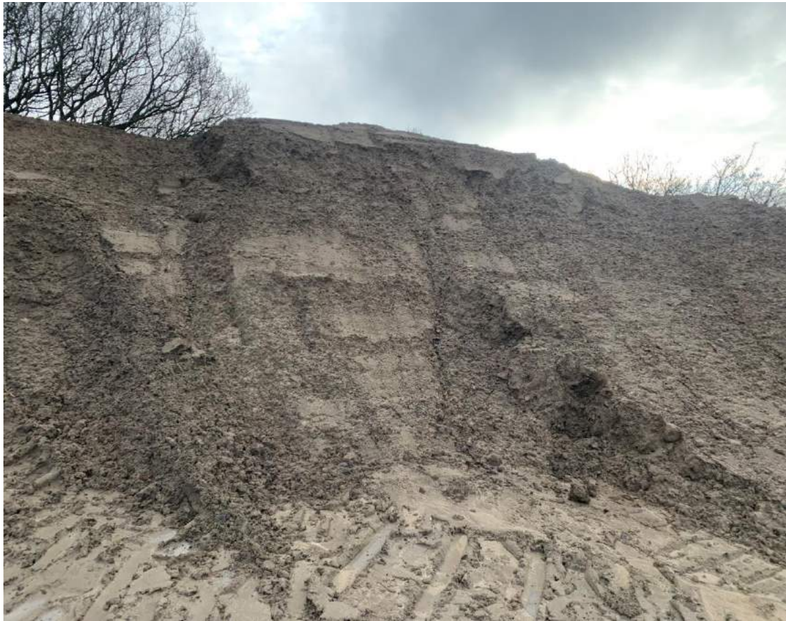
Plate 3 – Marchington Quarry, Glossop. NX Inspection 20 th March 2024
