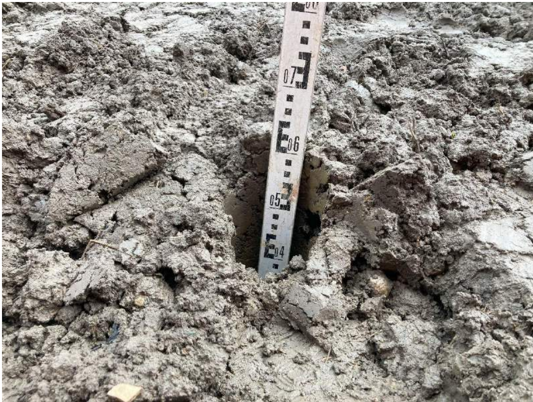
Plate 3 – Plot 1 front garden cover system GL to 0.60mbgl with 0.15m of topsoil.
