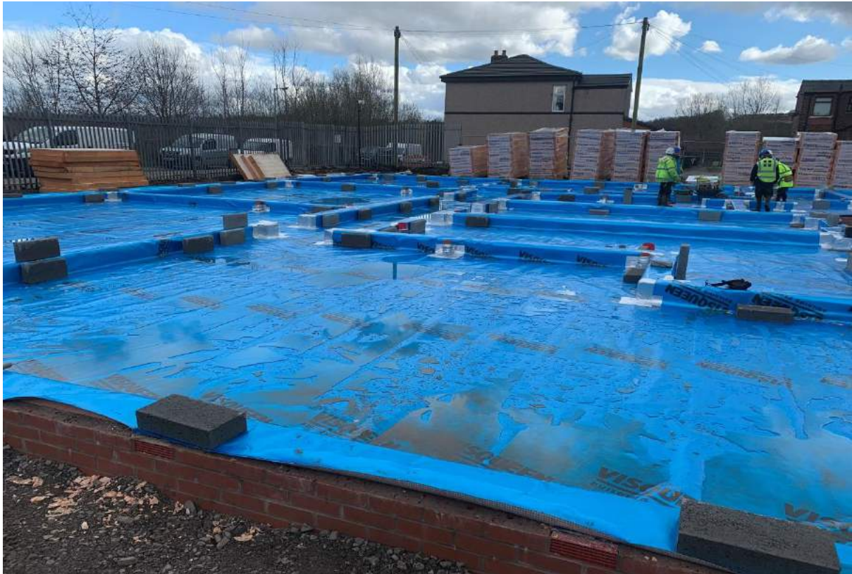
PLATE 1: Apt 1 to 20 with Full Visqueen Barrier Coverage
