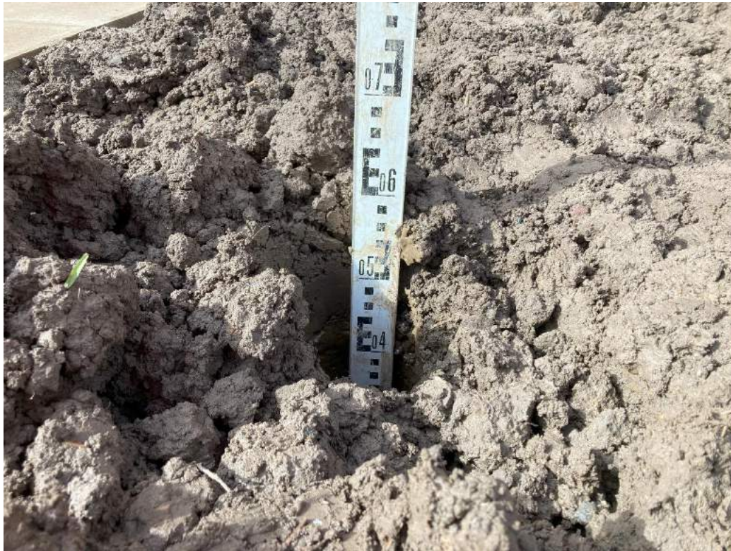
Plate 13 – Plot 3 front garden cover system GL to 0.60mbgl with 0.15m of topsoil.
