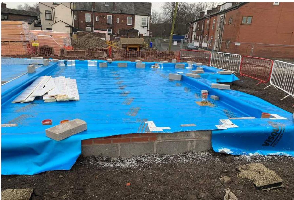
PLATE 1: Plot 1 with Full Visqueen Barrier Coverage
