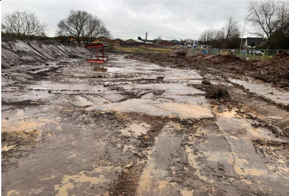
Plate 2 – Millar Homes Topsoil Source, Widnes. NX Inspection 1 st March 2024
