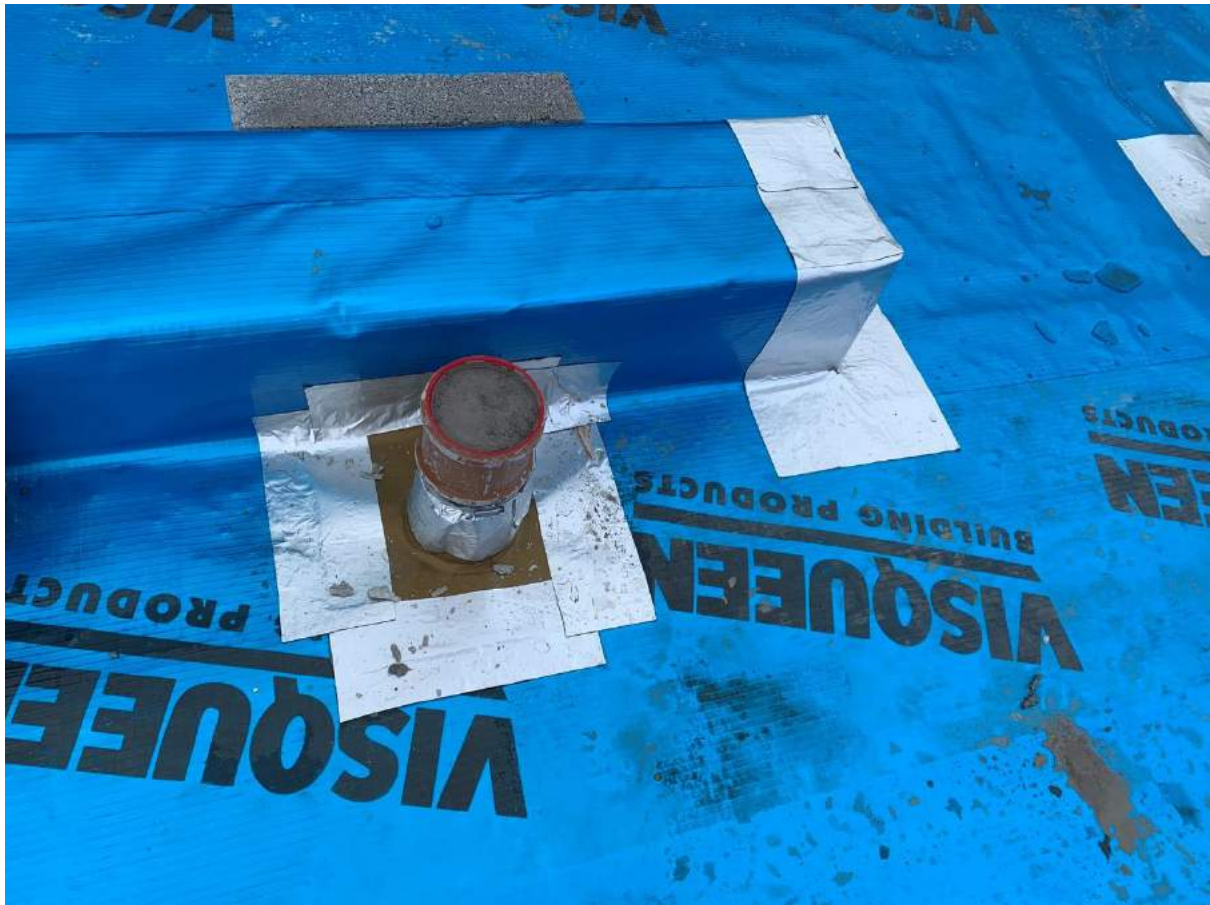
PLATE 4: Service Entry Detail Example
