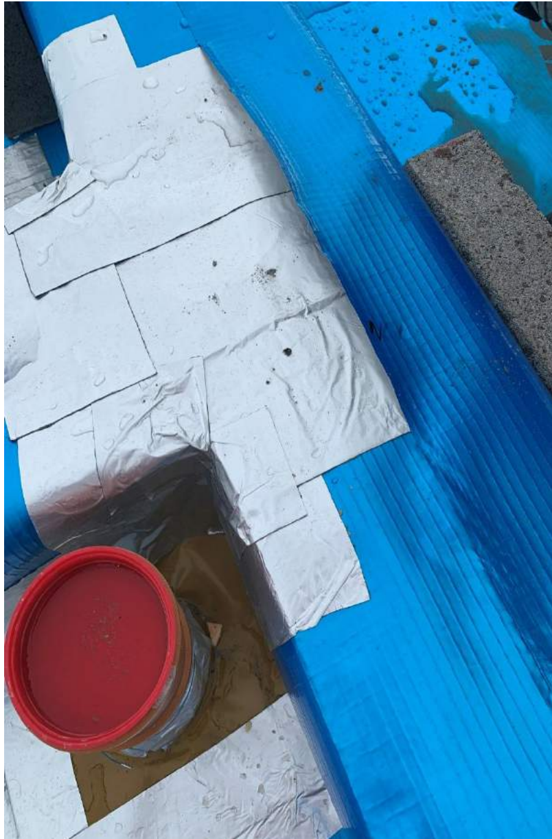
PLATE 3: NC1 Patch Repair
