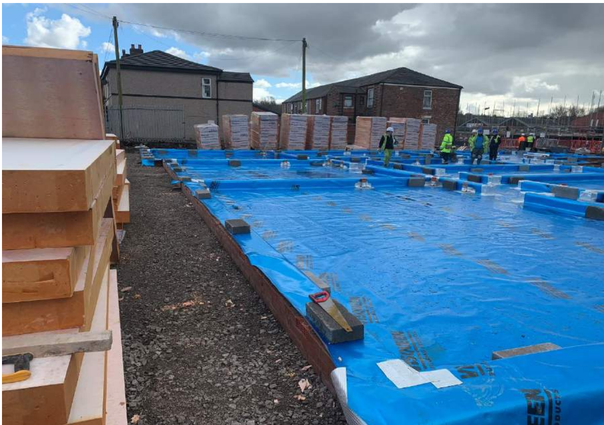
PLATE 2: Apt 1 to 20 with Full Visqueen Barrier Coverage
