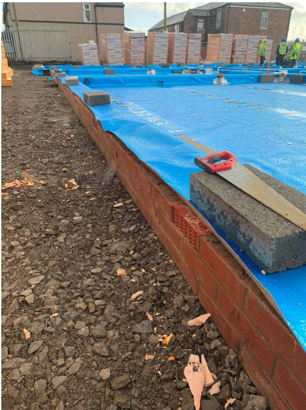
PLATE 8: Subfloor Venting on 2m to 3m centres
