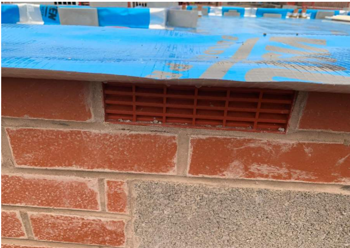
PLATE 8: Subfloor Venting on 2m centres
