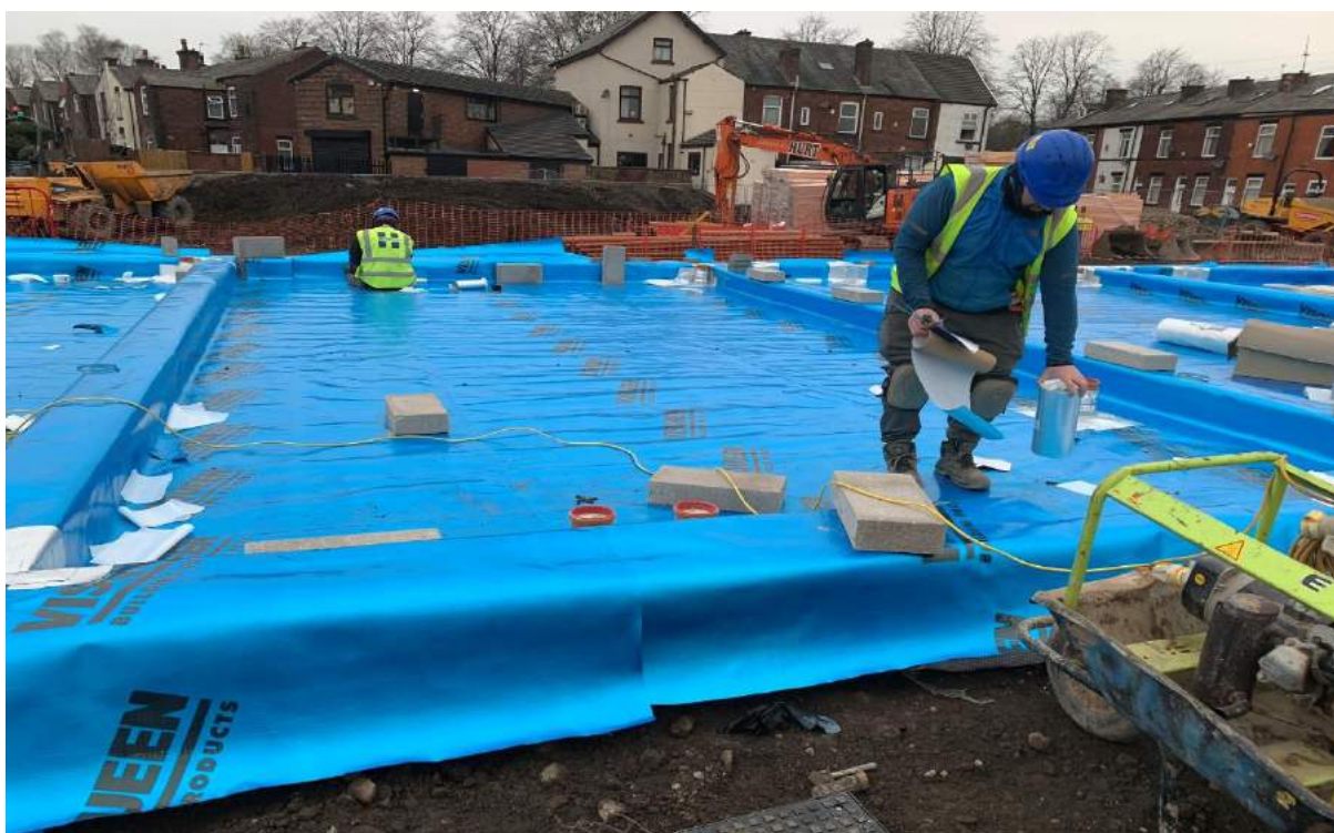
PLATE 4: Plot 6 with Full Visqueen Barrier Coverage
