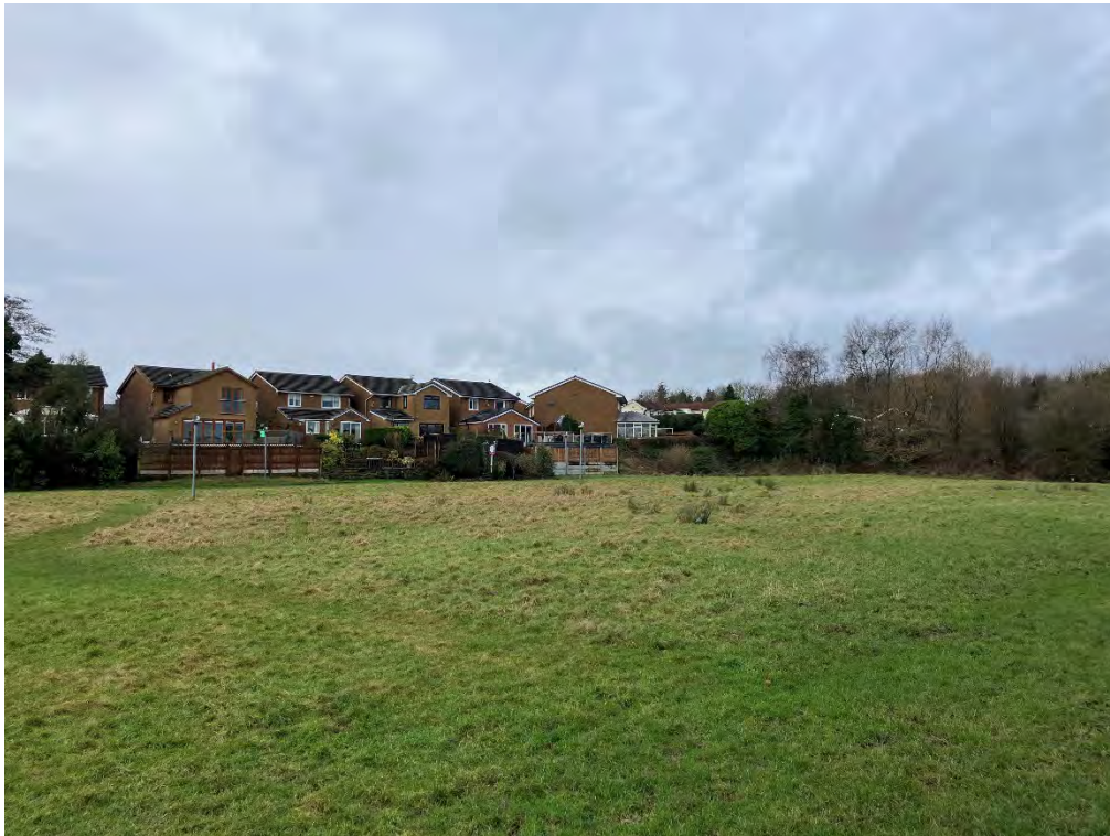
Plate 3: View of the rear gardens of Camden Close from the south-eastern side of The Delph showing fencing at numbers 14 and 10 as well as methane vents, facing north-west
