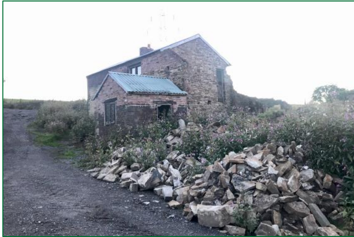
The building, looking southwest
