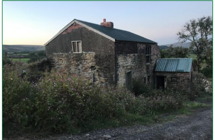
The building, looking northeast
