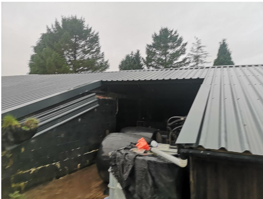
Plate 7 –eastern elevation, open access to the stable
