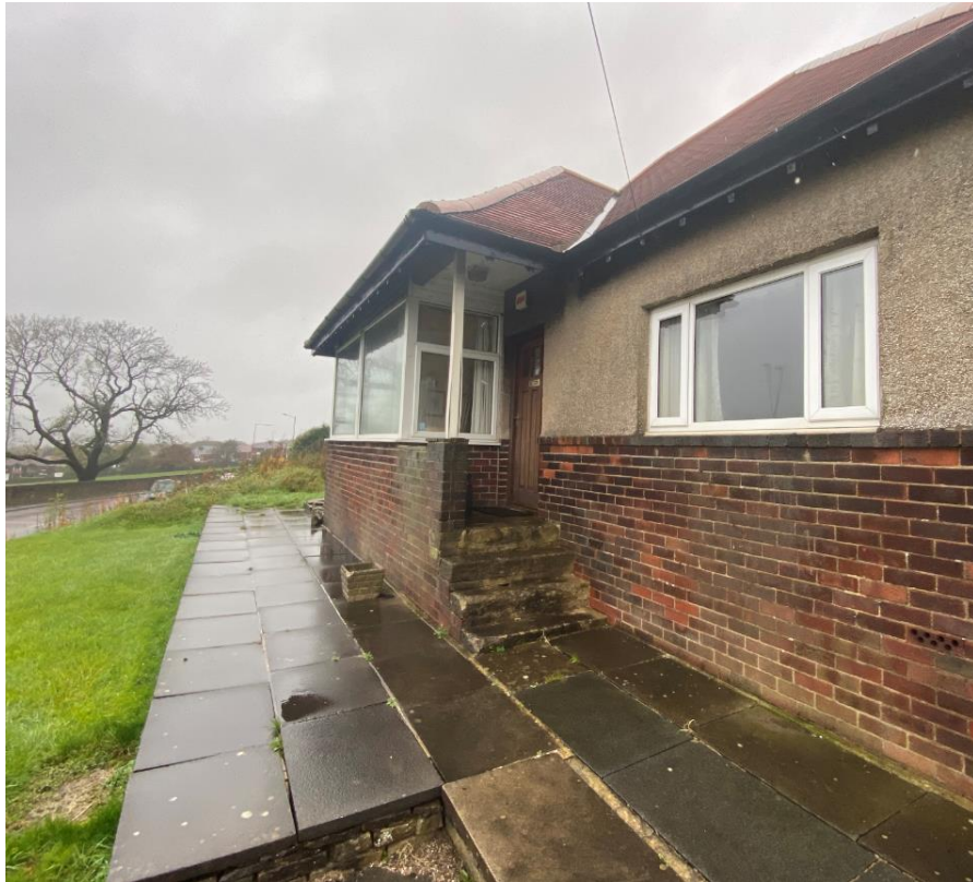
Photograph of Existing open porch area
