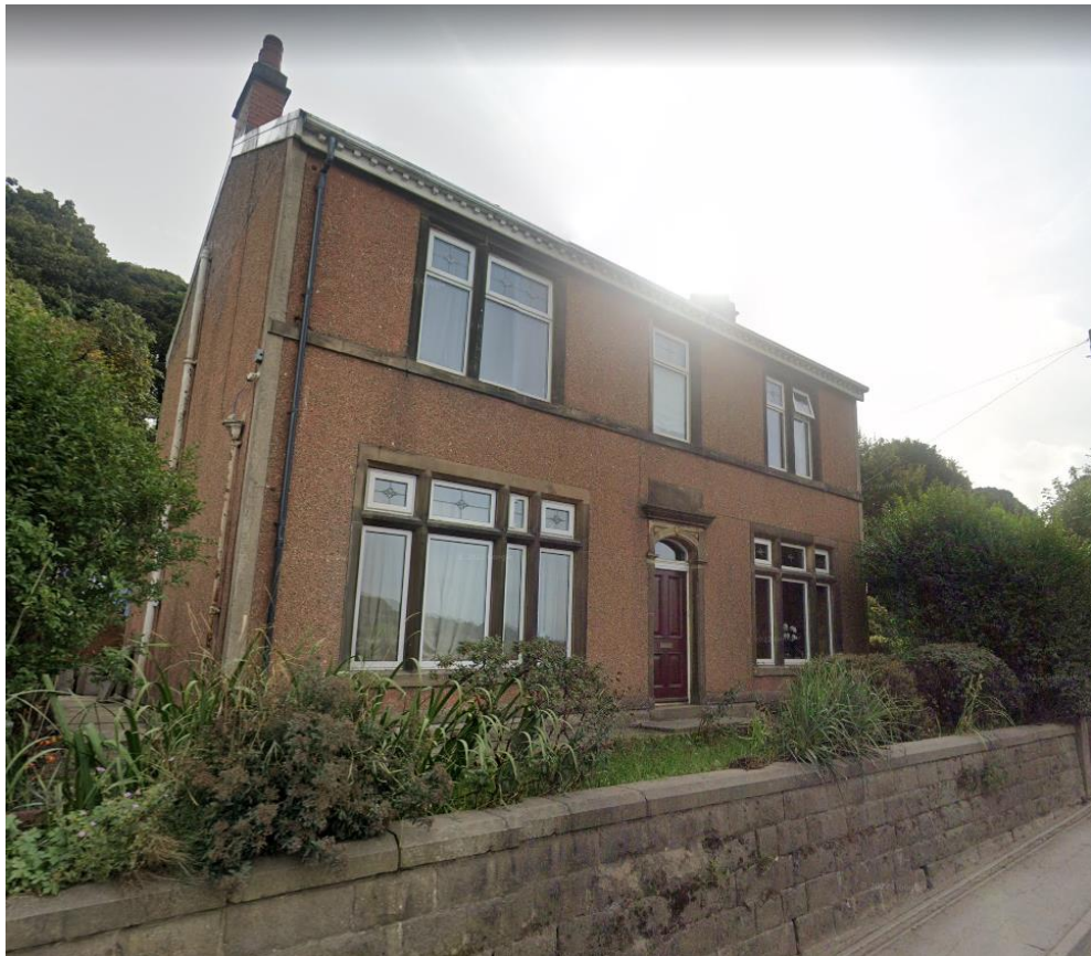
211 Manchester Road, a large 2 storey dwelling with Pebble dash render finish and stone Features with a slate roof.
