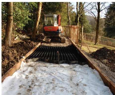
Fallbarrow Park, Windermere: CellWeb TRP® Installation
