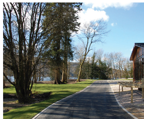
Fallbarrow Park, Windermere: Completed CellWeb TRP® Installation
