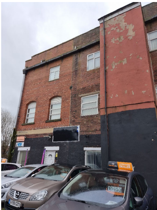
Photo 8 - North gable elevation
