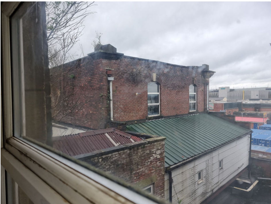
Photo 6 – View looking towards Fountain Street from 2 nd floor
