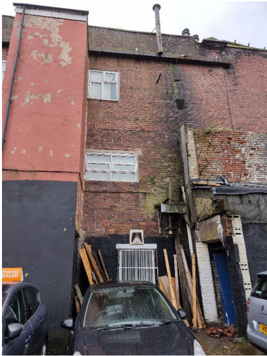
Photo 7 – North gable elevation
