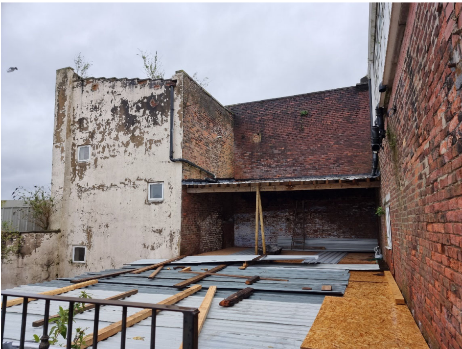
Photo 12 – South elevation roof terrace
