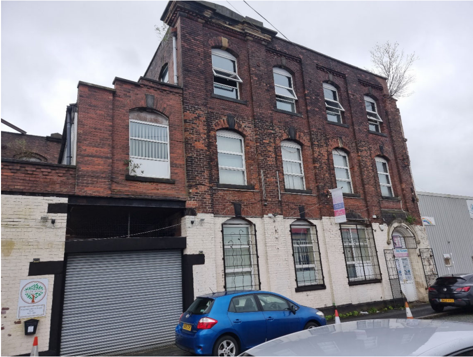
Photo 3 – Fountain Street elevation
