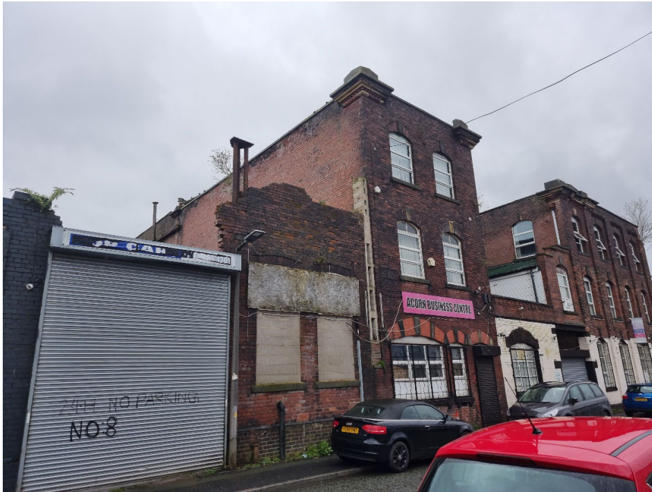
Photo 1 – Fountain Street elevation
