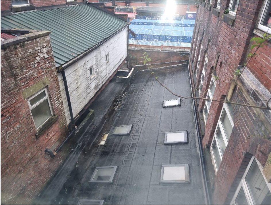
Photo 5 – View looking towards Fountain Street from 2 nd floor
