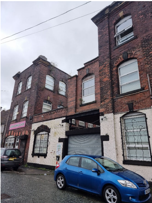
Photo 4 – Fountain Street elevation
