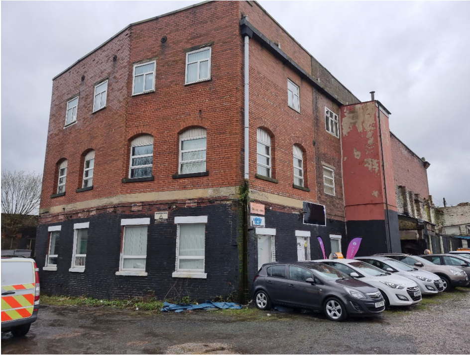
Photo 9 – East gable elevation
