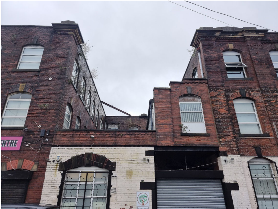
Photo 2 – Fountain Street elevation
