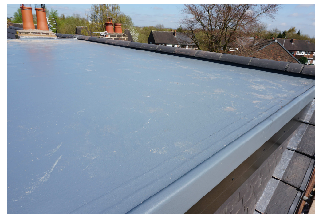
Typical Fibreglass Finish to New Flat Roof
