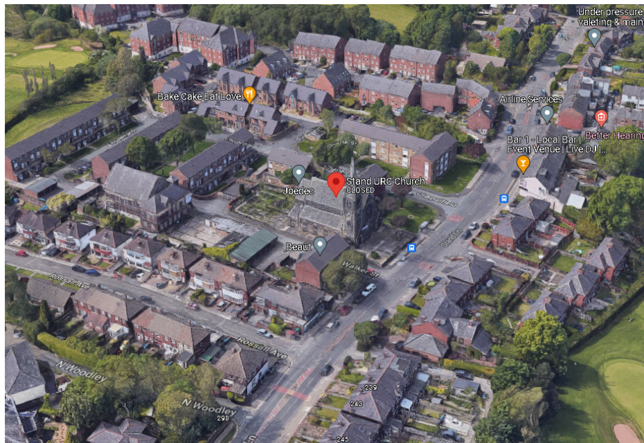
Image 01: the existing church building and its site setting.
