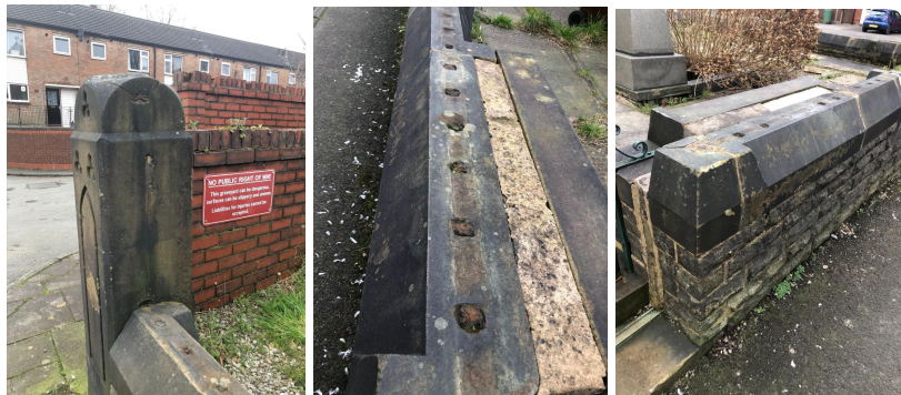
Image 02: Remnants of previously installed perimeter railings
