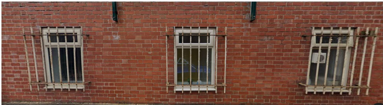
Figure 14 – Windows to be replaced on Back Rock
