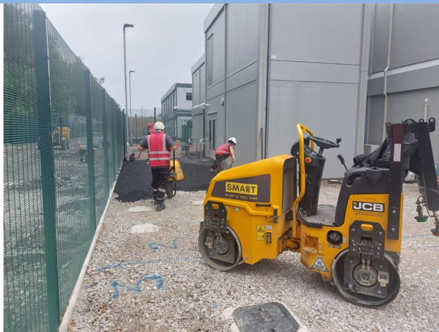
Photograph 1 – View of capping layer prior to laying of tarmac of MUGA pitch
