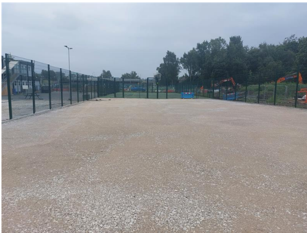
Photograph 1 – View of capping layer prior to laying of tarmac of MUGA pitch
