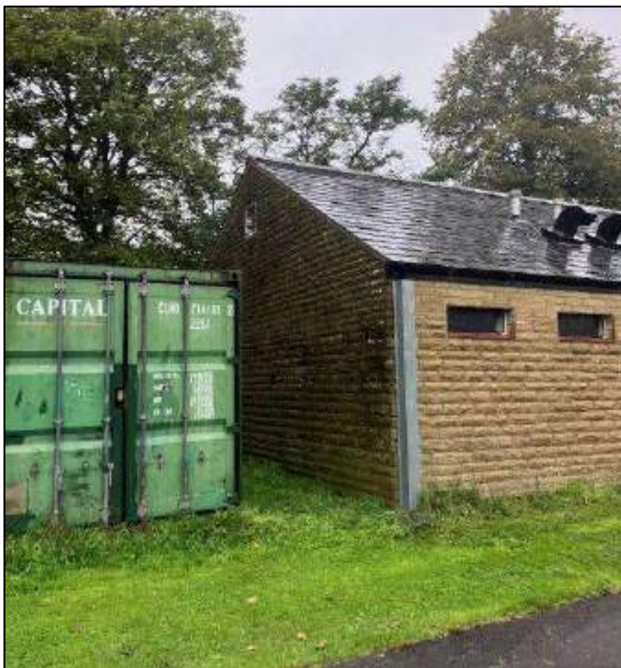
Figure 2-D: Photograph showing area of proposed pavilion extension.
