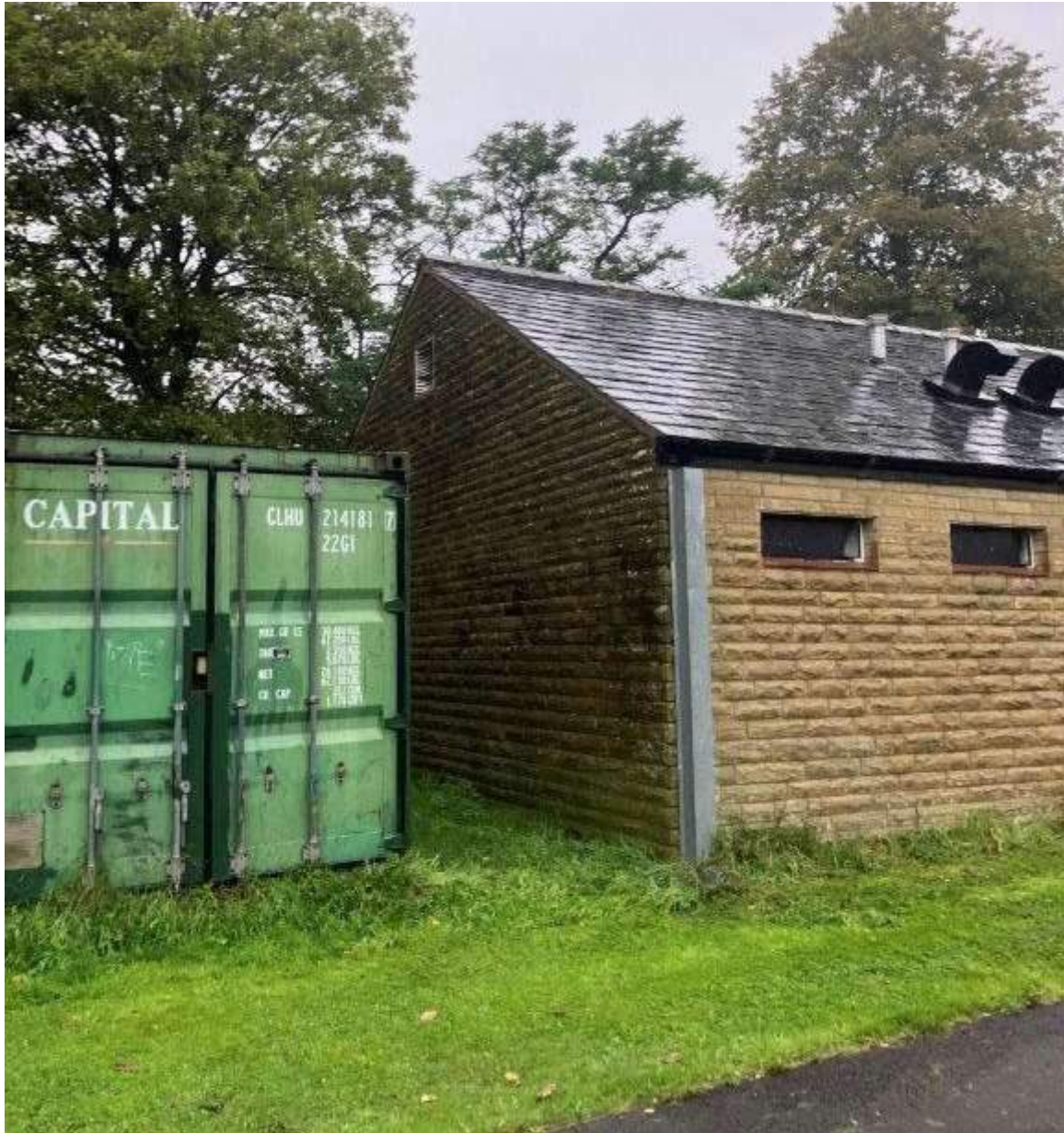
Photo 3: Photograph showing area of proposed pavilion extension.
