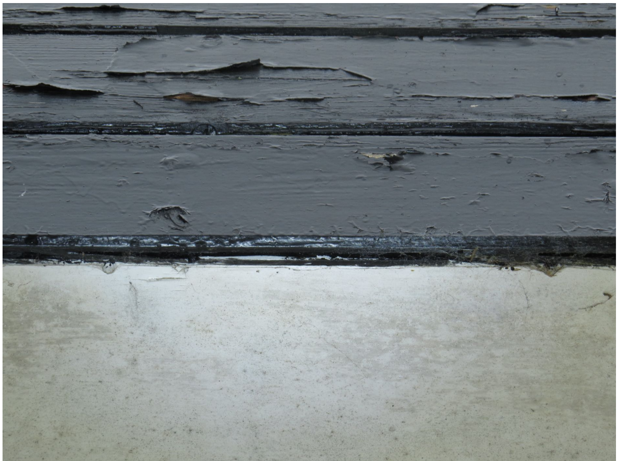
4 – Fascia boards and soffits at the eaves are fixed tightly against brickwork.
