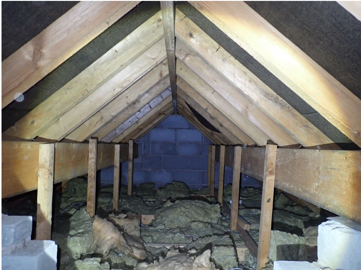
3.2a – The roof void.
