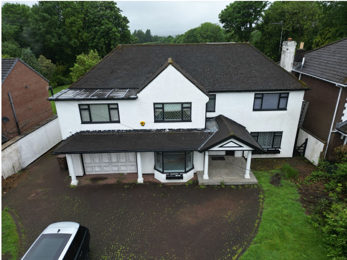
3.1a – The front of the house.
