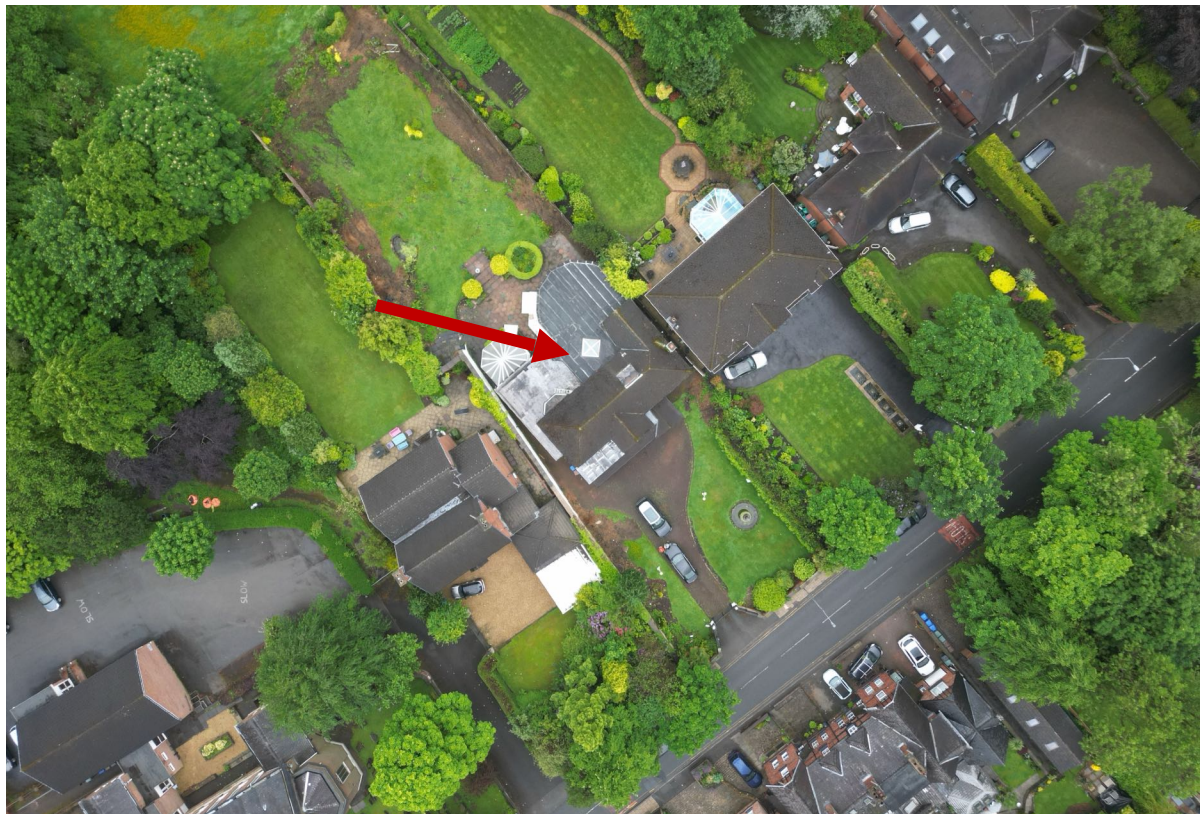
1.6b – 54 Ringley Road – aerial photograph.
