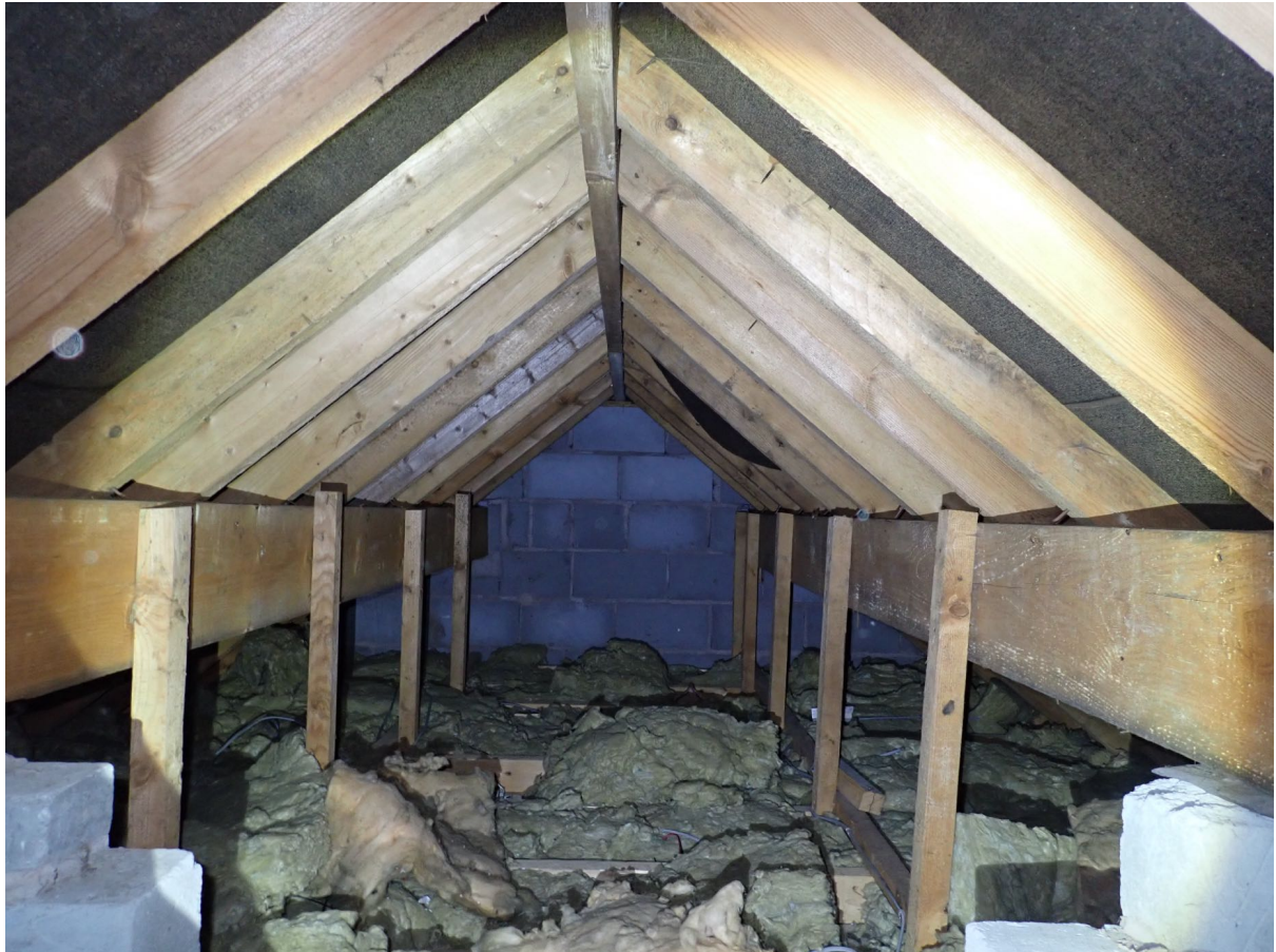
9 – The house has loft voids at the gables and crawl spaces at the eaves.
