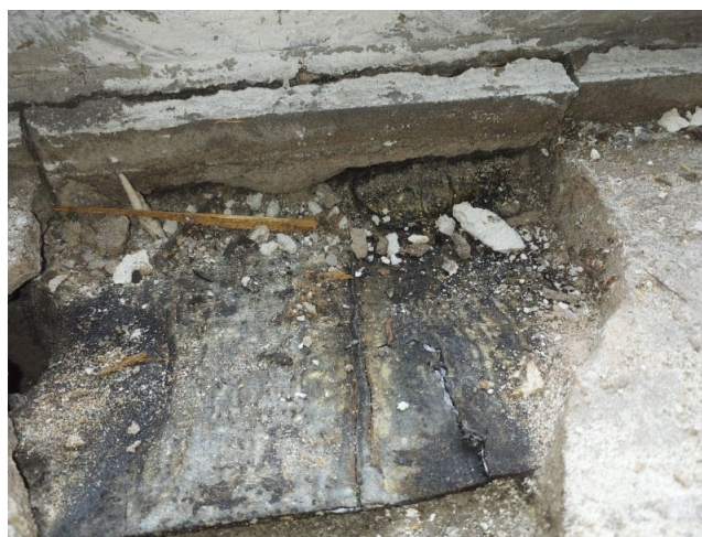
Sample No: 23/5/B/18/SAW11 External Window reveals Bitumen vapour barrier No Asbestos Detected
