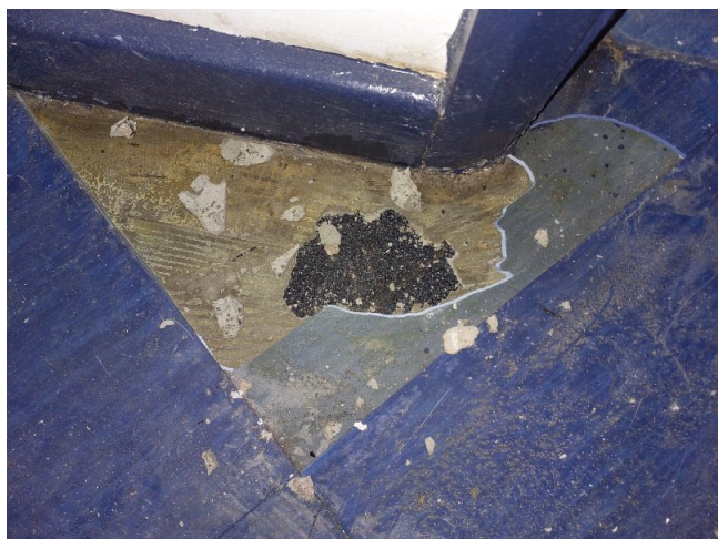
Sample No: Refer to Sample 23/5/B/18/SAW5 1.02 Circulation Floor below screed Bitumen adhesive residuals containing: Chrysotile
