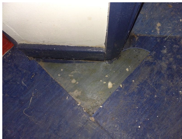
Sample No: Refer to Sample 23/5/B/18/SAW4 1.02 Circulation Bottom layer of floor covering Vinyl floor covering No Asbestos Detected
