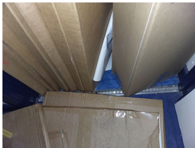
Sample No: Refer to Sample 23/5/B/18/SAW4 1.03 Cupboard Bottom layer of floor covering Vinyl floor covering No Asbestos Detected
