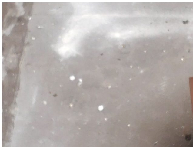
Sample No: 23/5/B/18/SAW13 External Roof Core sample No Asbestos Detected
