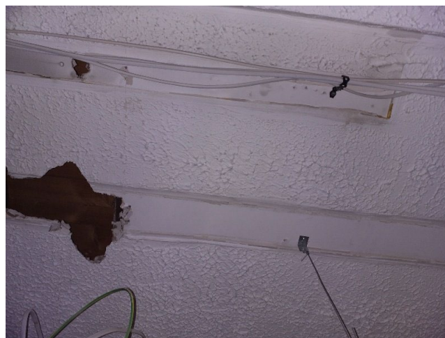
Sample No: 23/5/B/18/SAW6 1.04 Staff kitchen Ceiling void Textured coating to plasterboard ceiling No Asbestos Detected
