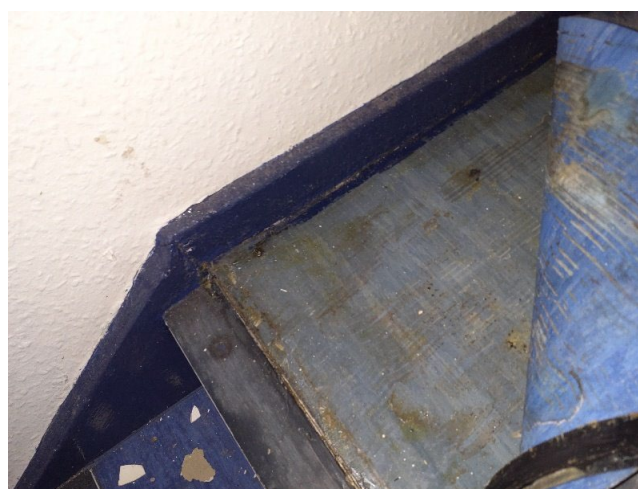
Sample No: 23/5/B/18/SAW4 1.01 Landing Bottom layer of floor covering Vinyl floor covering No Asbestos Detected
