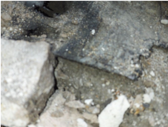
Sample No: Refer to Sample 23/5/B/18/SAW1 External Window reveals Bitumen vapour barrier No Asbestos Detected
