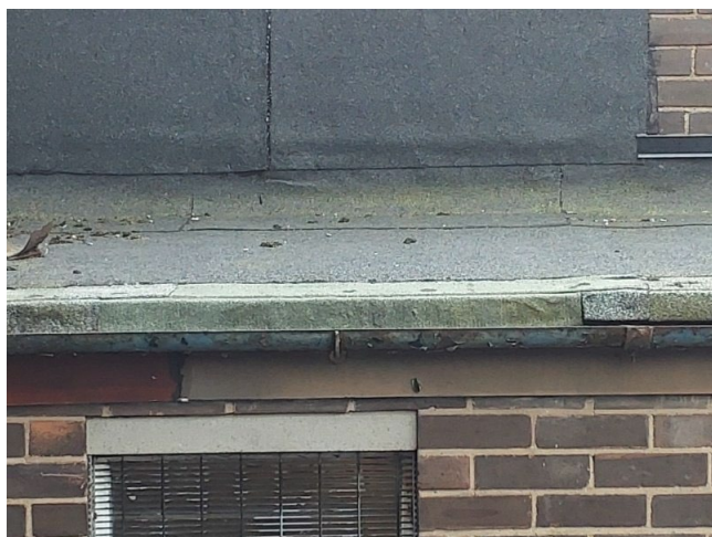
Sample No: 23/5/B/18/SAW12 External Roof Core sample No Asbestos Detected
