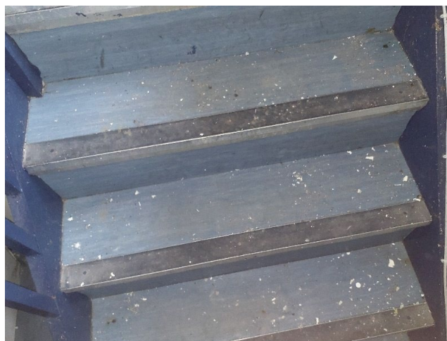
Sample No: Refer to Sample 23/5/B/18/SAW3 1.08 Stairwell Staircase Nose edgings No Asbestos Detected
