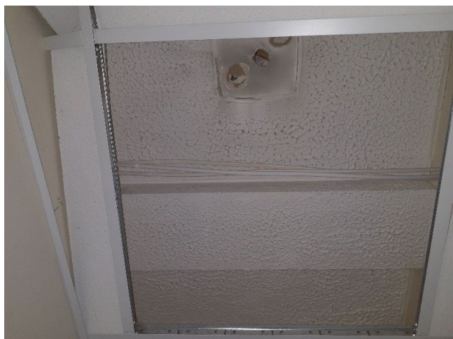
Sample No: Refer to Sample 23/5/B/18/SAW6 1.05 Toilet and lobby Ceiling void Textured coating to plasterboard ceiling No Asbestos Detected
