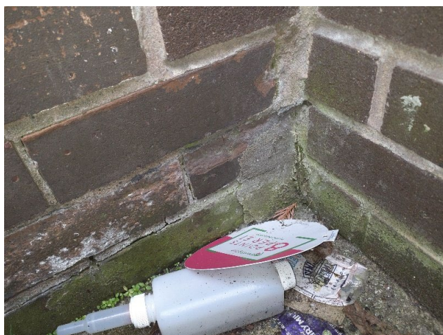
Sample No: 23/5/B/18/SAW10 External Damp proof course Bitumen damp proof No Asbestos Detected
