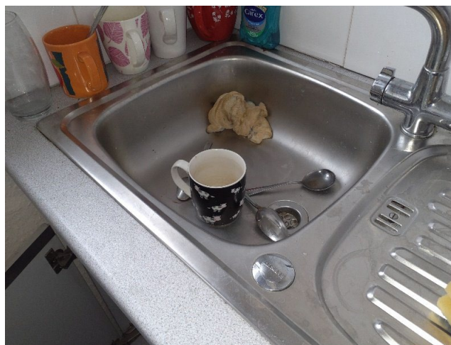
Sample No: 23/5/B/18/SAW8 2.02 Kitchen Sink Sink pad No Asbestos Detected
