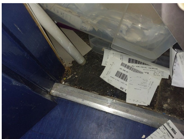
Sample No: Refer to Sample 23/5/B/18/SAW5 1.07 Cupboard Floor below screed Bitumen adhesive residuals containing: Chrysotile
