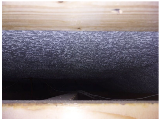
Sample No: 23/5/B/18/SAW2 G.03 Customer toilet Ceiling void Textured coating to plasterboard ceiling No Asbestos Detected
