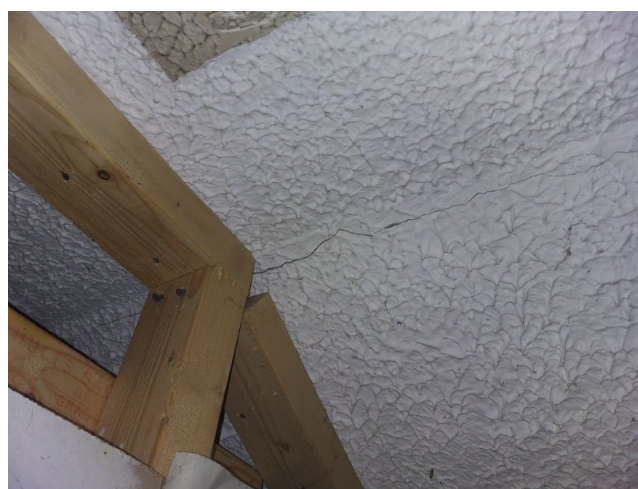
Sample No: Refer to Sample 23/5/B/18/SAW2 G.05 Rear circulation Ceiling void Textured coating to plasterboard ceiling No Asbestos Detected
