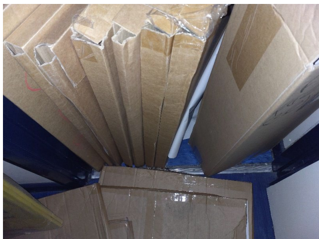
Sample No: Refer to Sample 23/5/B/18/SAW5 1.03 Cupboard Floor below screed Bitumen adhesive residuals containing: Chrysotile
