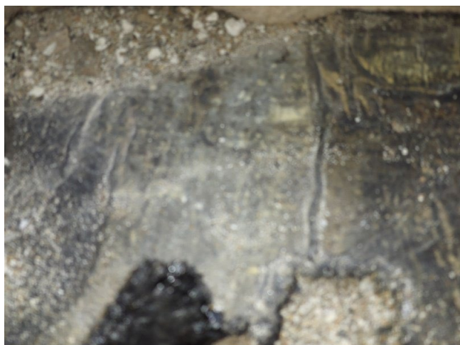
Sample No: Refer to Sample 23/5/B/18/SAW17 External Window reveals Bitumen vapour barrier No Asbestos Detected
