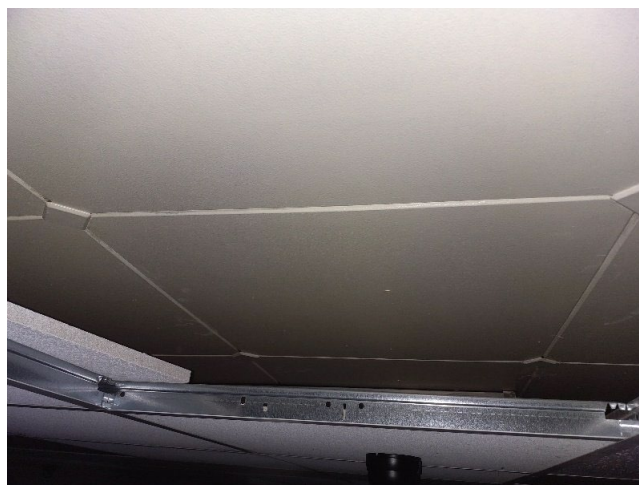
Sample No: 23/5/B/18/SAW14 G.01 Shop area Ceiling void Plasterboard ceiling tiles No Asbestos Detected
