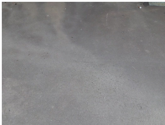
Sample No: 23/5/B/18/SAW19 External Roof Core sample No Asbestos Detected
