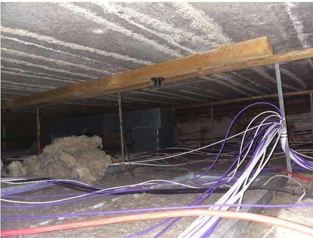
Sample No: Refer to Sample 23/4/B/25/JPS5 G.02 Retail Sales Floor Ceiling Void Warm Air Ductwork Joints Mastic No Asbestos Detected
