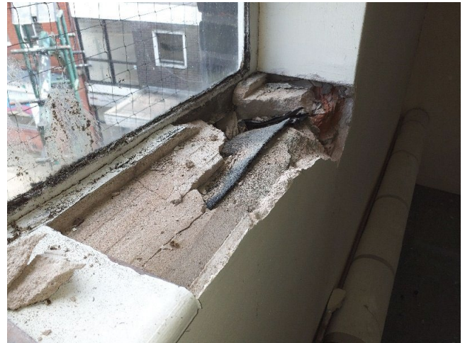
Sample No: 23/4/B/25/JPS18 2.01 Stairs / Storage Area Window Cavity Bitumen Vapour Barrier No Asbestos Detected
