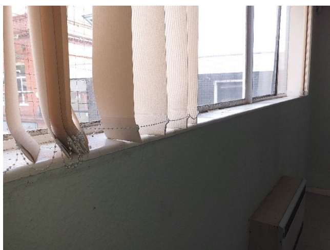
Sample No: Refer to Sample 23/4/B/25/JPS14 1.06 Kitchen Window Cavity Bitumen Vapour Barrier No Asbestos Detected
