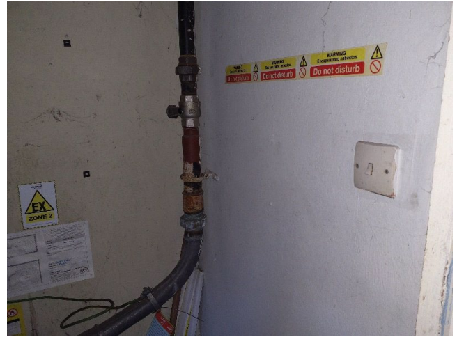
Sample No: Refer to Sample 23/4/B/25/JPS7 G.05 Store Room Internal Linings to Store Room Walls Insulating Board containing: Amosite & Chrysotile
