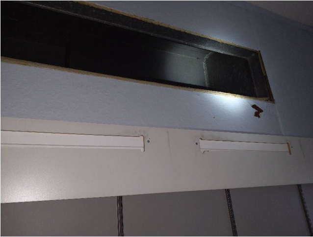
Sample No: 23/4/B/25/JPS5 G.02 Retail Sales Floor Warm Air Ductwork Joints Mastic No Asbestos Detected
