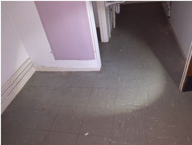
Sample No: Refer to Sample 23/4/B/25/JPS11 1.03 Toilets Floor Area Vinyl Floor Tiles No Asbestos Detected
