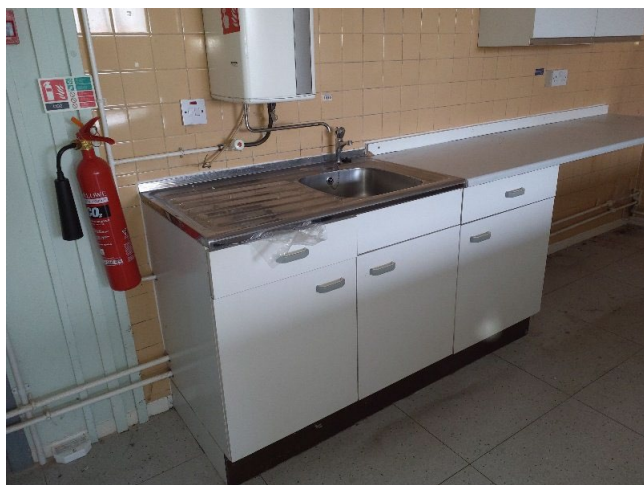
Sample No: 23/4/B/25/JPS15 1.06 Kitchen Sink Bitumen Pad No Asbestos Detected
