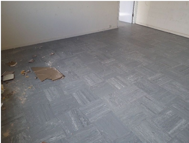
Sample No: 23/4/B/25/JPS17 2.01 Stairs / Storage Area Floor Area Vinyl Floor Tiles No Asbestos Detected
