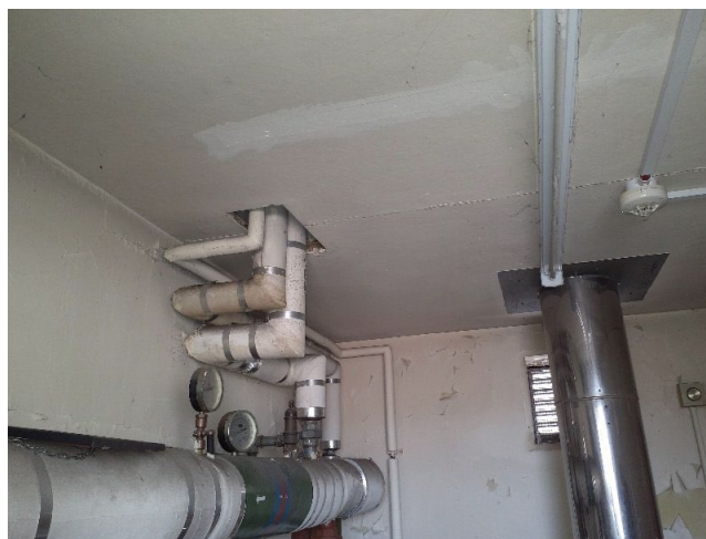
Sample No: 23/4/B/25/JPS20 2.03 Boiler Room Ceiling & Upstand Insulating Board No Asbestos Detected
