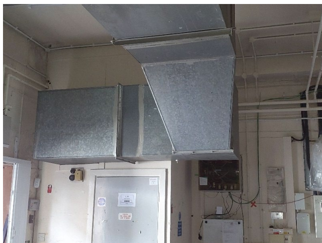
Sample No: Refer to Sample 23/4/B/25/JPS5 G.03 Warehouse Warm Air Ductwork Joints Mastic No Asbestos Detected
