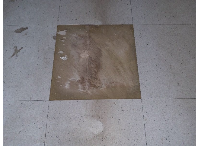
Sample No: Refer to Sample 23/4/B/25/JPS1 G.02 Retail Sales Floor Floor Area Below Vinyl Floor Tiles Terrazzo Flooring Infill No Asbestos Detected
