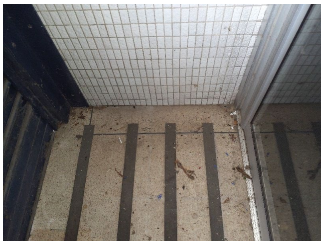
Sample No: 23/4/B/25/JPS1 G.01 Entrance Lobby Floor Area Terrazzo Flooring Infill No Asbestos Detected
