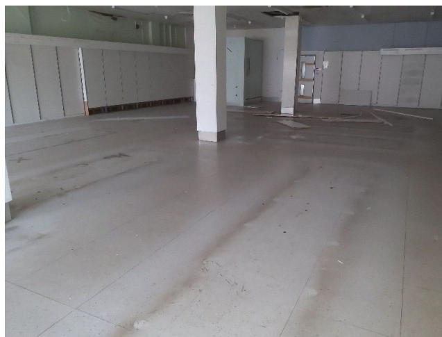
Sample No: 23/4/B/25/JPS2 G.02 Retail Sales Floor Floor Area Vinyl Floor Tiles No Asbestos Detected
