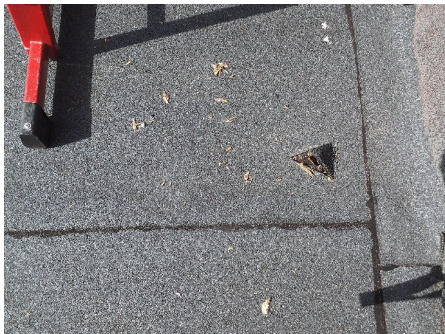
Sample No: 23/4/B/25/JPS21 External Flat Roof Area Core Sample No Asbestos Detected
