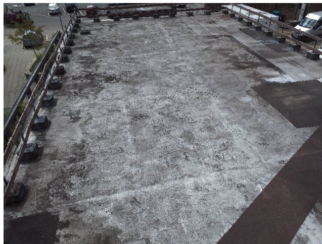
Sample No: 23/4/B/25/JPS22 External Flat Roof Area Core Sample No Asbestos Detected
