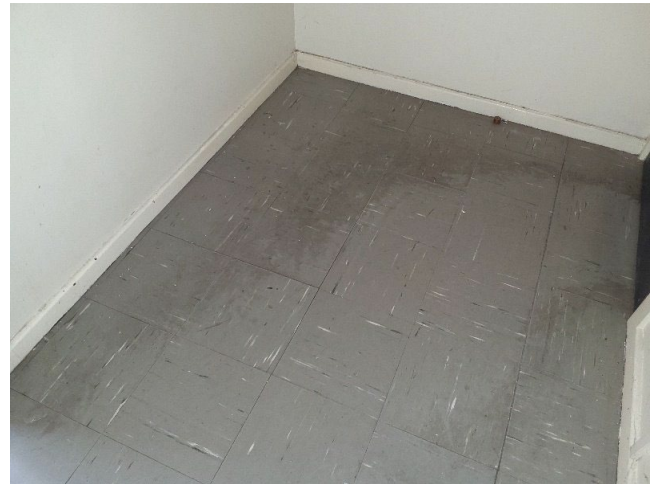
Sample No: Refer to Sample 23/4/B/25/JPS11 1.04 Circulation Area Floor Area Vinyl Floor Tiles No Asbestos Detected
