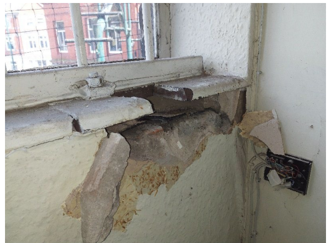
Sample No: 23/4/B/25/JPS14 1.05 Office Window Cavity Bitumen Vapour Barrier No Asbestos Detected
