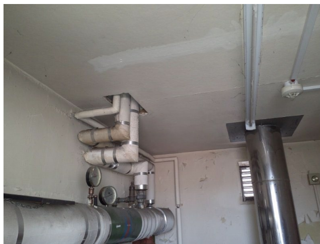
Sample No: Refer to Sample 23/4/B/25/JPS20 3.01 Tank Room Pipework Upstand Insulating Board No Asbestos Detected
