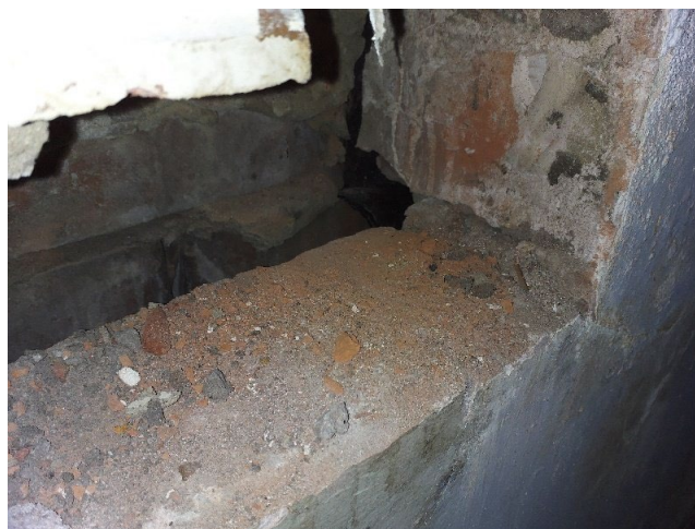
Sample No: 23/4/B/25/JPS8 G.03 Warehouse Window Cavity Bitumen Vapour Barrier No Asbestos Detected
