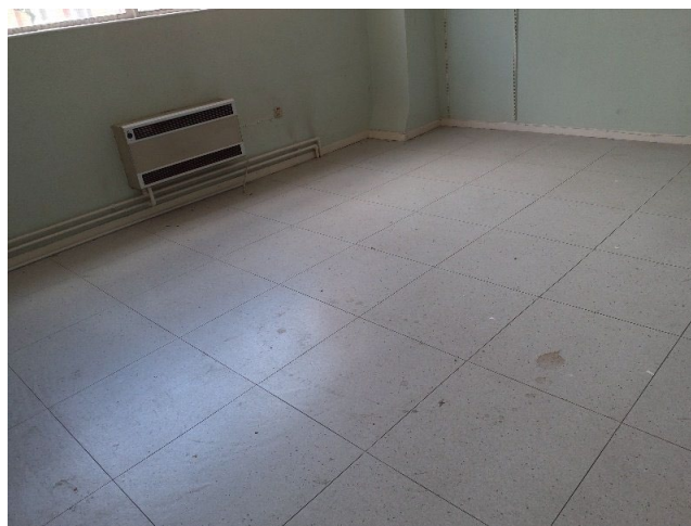
Sample No: Refer to Sample 23/4/B/25/JPS2 1.06 Kitchen Floor Area Vinyl Floor Tiles No Asbestos Detected
