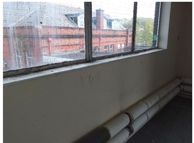
Sample No: Refer to Sample 23/4/B/25/JPS18 2.02 Store Room Window Cavity Bitumen Vapour Barrier No Asbestos Detected
