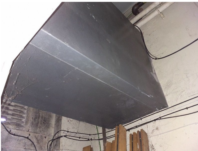
Sample No: Refer to Sample 23/4/B/25/JPS5 G.05 Store Room Warm Air Ductwork Joints Mastic No Asbestos Detected
