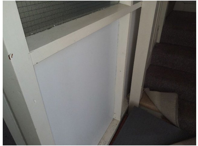
Sample No: 23/4/B/18/JPS7 1.01 Entrance Lobby Combination Frame Spandrel Panels Composite Board No Asbestos Detected
