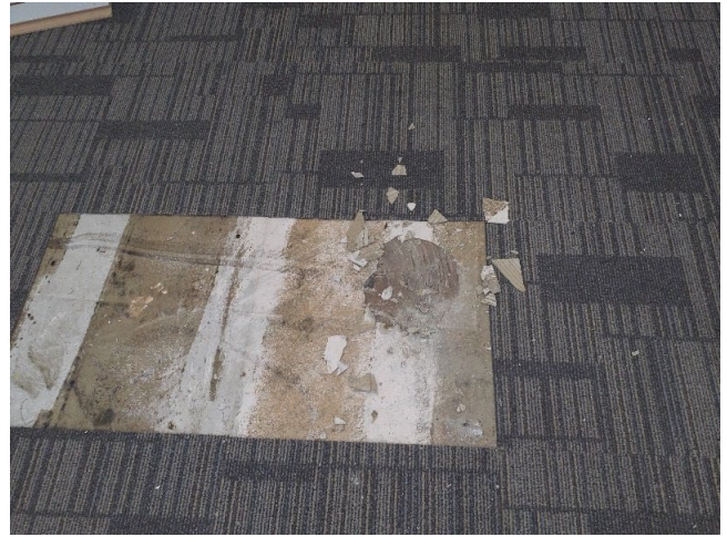
Sample No: 23/4/B/18/JPS2 G.01 Retail Area Floor Area (Below Carpet & Screed) Floor Tiles and Bitumen Adhesive No Asbestos Detected
