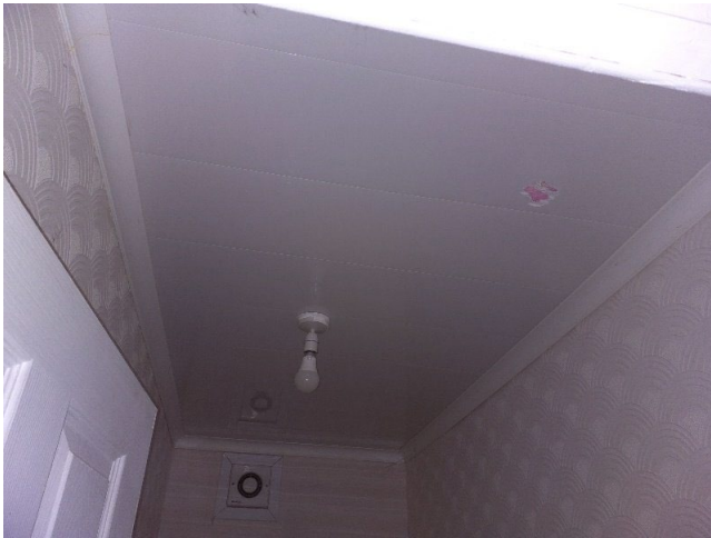
Sample No: Refer to Sample 22/12/B/13/MAC1 G.03 Toilet Ceiling Fibreboard No Asbestos Detected
