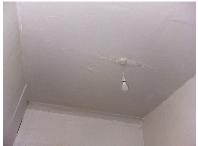
Sample No: Refer to Sample 22/12/B/13/MAC1 G.02 Store room Ceiling Fibreboard No Asbestos Detected
