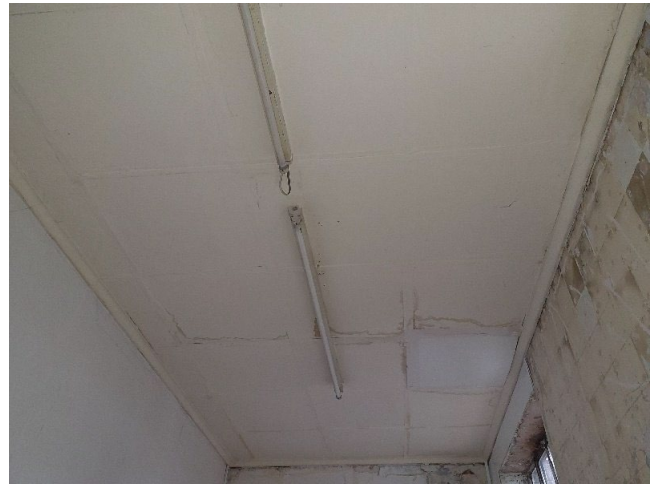
Sample No: Refer to Sample 22/12/B/13/MAC1 G.06 Kitchen Ceiling Fibreboard No Asbestos Detected
