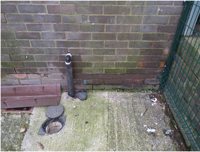
Sample No: 22/12/B/13/MAC3 External Walls Bitumen DPC No Asbestos Detected
