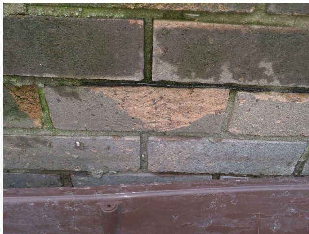
Sample No: 22/12/B/13/SAW4 External Damp proof course Bitumen Layer No Asbestos Detected
