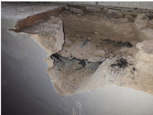
Sample No: 22/12/B/13/SAW3 External Windows Bitumen vapour barrier to wall cavities No Asbestos Detected
