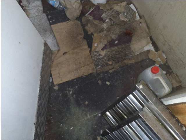
Sample No: Refer to Sample 22/12/B/13/SAW2 1.03 Toilet Floor
