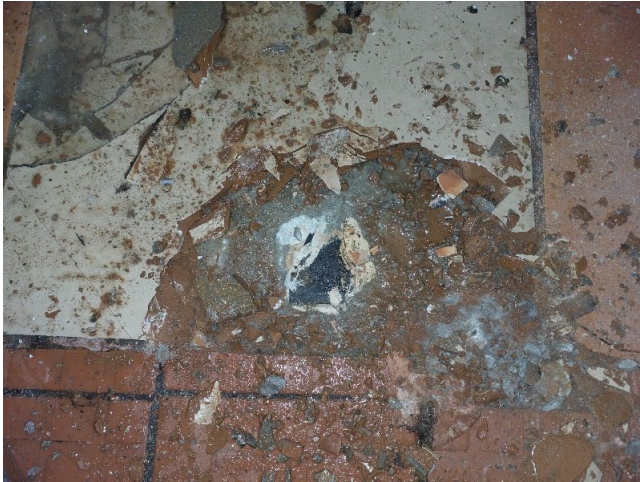
Sample No: Refer to Sample 22/12/B/13/SAW1 G.02 Food prep area Floor beneath screed Bitumen residuals containing: Chrysotile
