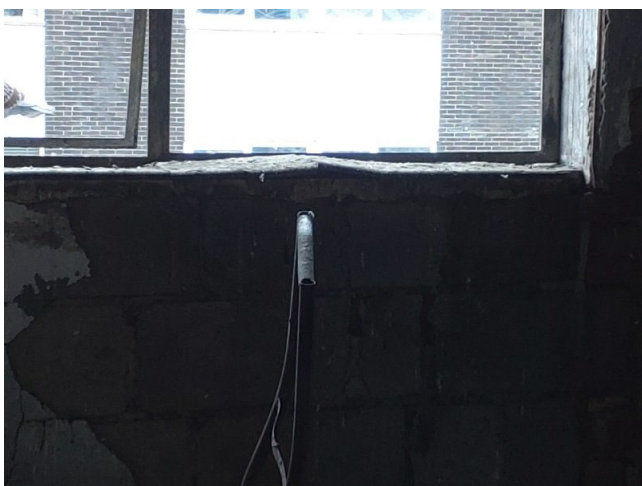
Sample No: Refer to Sample 22/12/B/13/SAW3 External Windows Bitumen vapour barrier to wall cavities No Asbestos Detected
