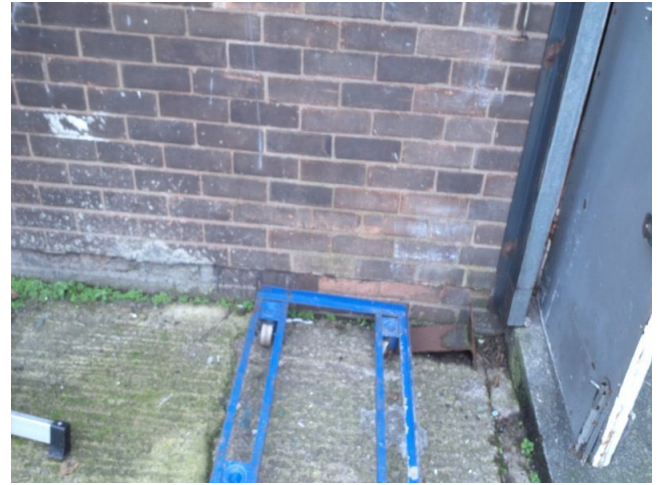
Sample No: 22/12/B/13/DAB13 External Damp proof course Bitumen Layer No Asbestos Detected
