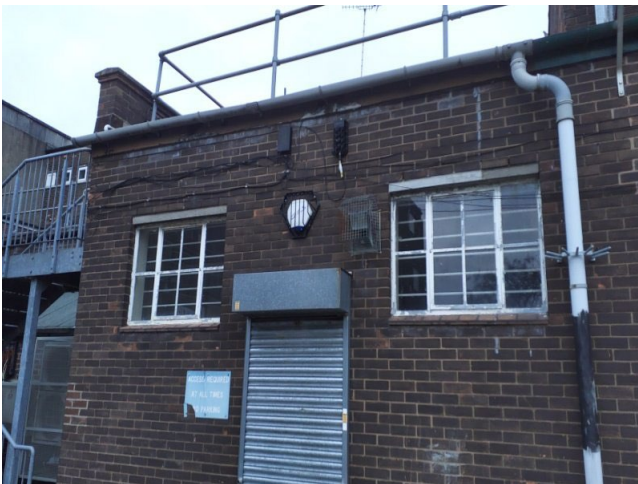
Sample No: Refer to Sample 22/12/B/13/DAB12 External Below windowsill and frames Bitumen vapor barrier No Asbestos Detected
