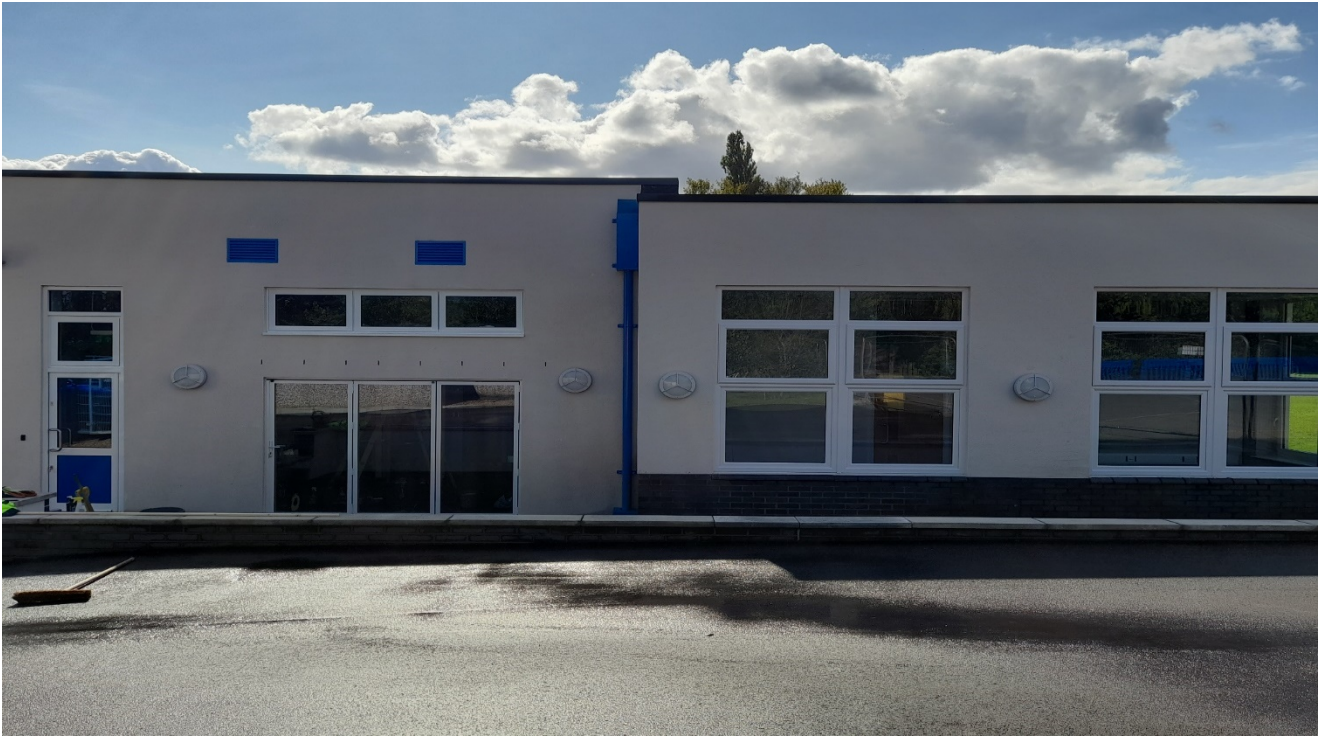
PHOTO 1: Existing rear Bi-fold doors ( 3 sections) the proposed location of the new canopy
