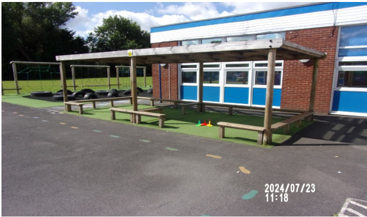
PHOTO 3: Previous open sided timber (stained) gazebo ( longer 7.5 m side view) put in place approximately 4 years ago, located alongside the early years playground. The main framing has bench type seating for teaching use in warm weather with an artificial inner grass floor for sitting -on.
