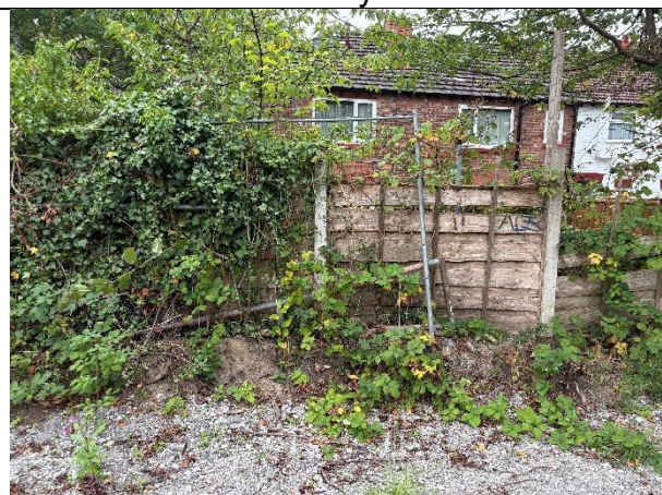
Photo 4: Extension of the bare ground habitat along the southeastern boundary.
