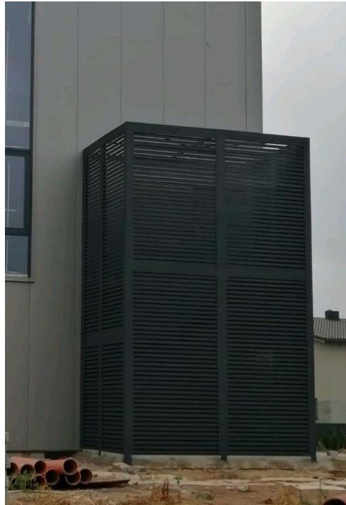
Fig's 14 and 15 Examples of similar style permeable cladding with flow of natural light and visual flow through cladding
