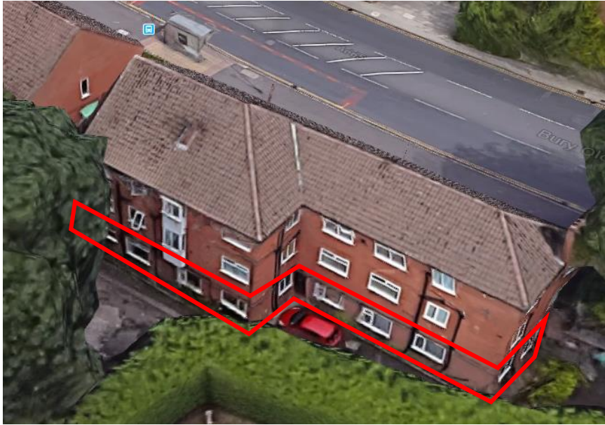
Fig 4. Picture showing location of flats at lower ground floor level
