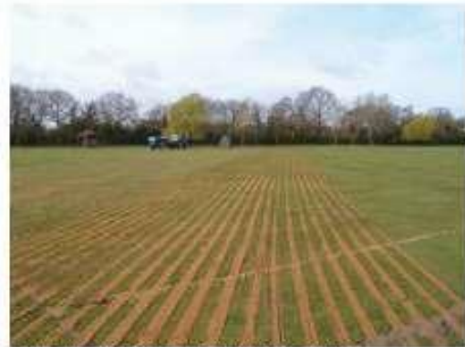
Sand grooves installed at 260 mm centres
