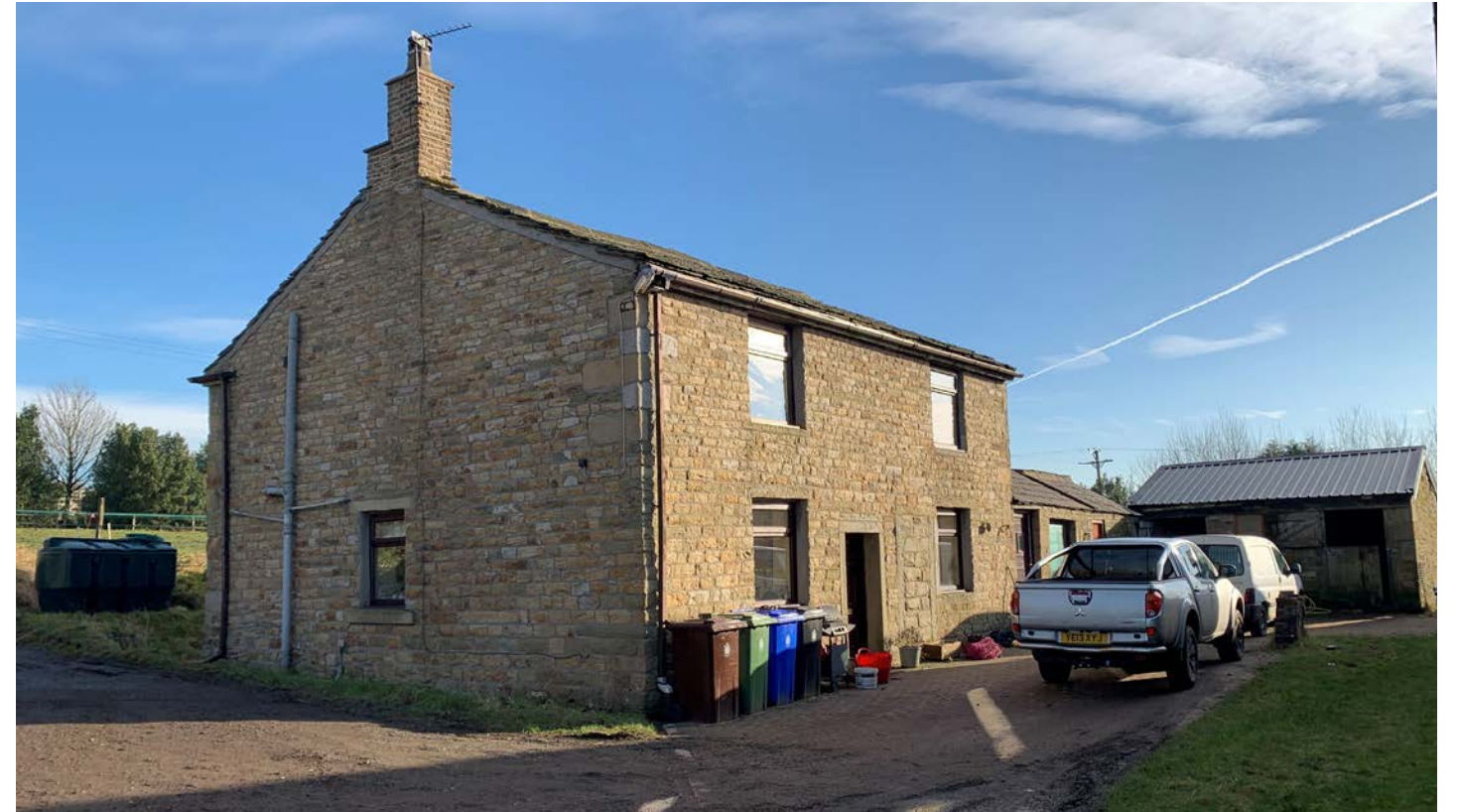
Above: Existing House - Front (Faces Dry Gap Barn)
