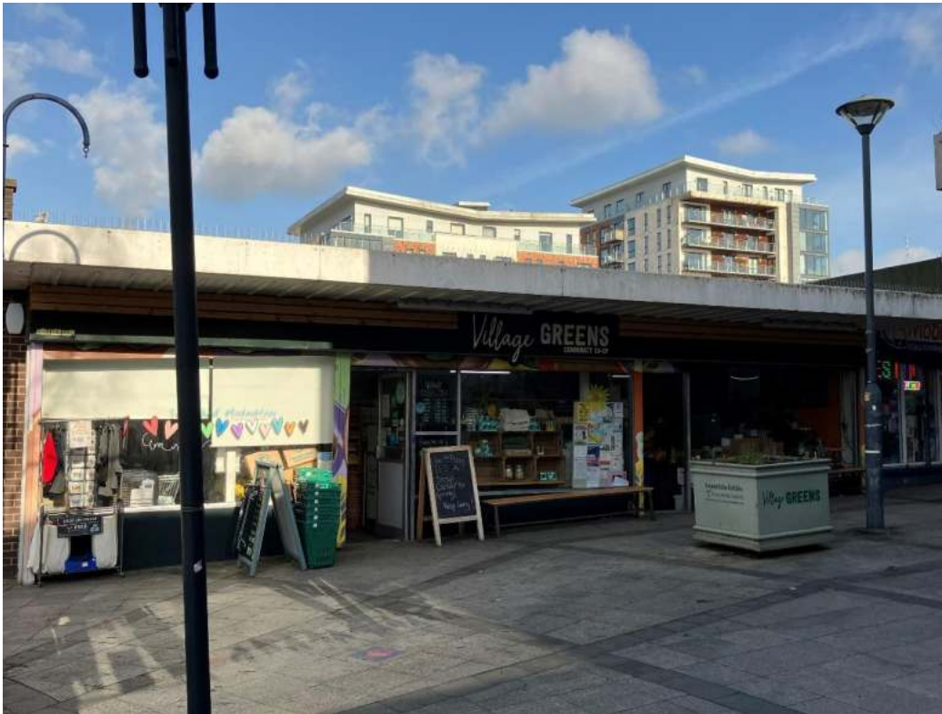
Single storey retail units at west end access to shopping centre
