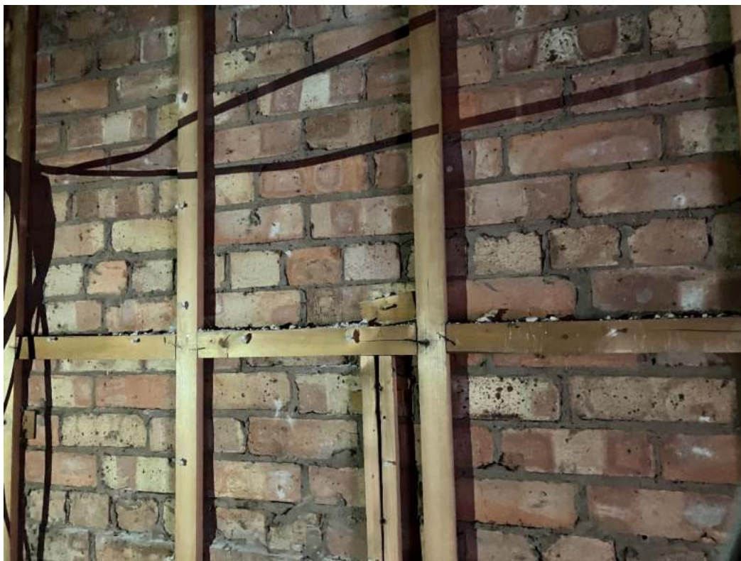
Exposed party wall after wall finishes stripped out
