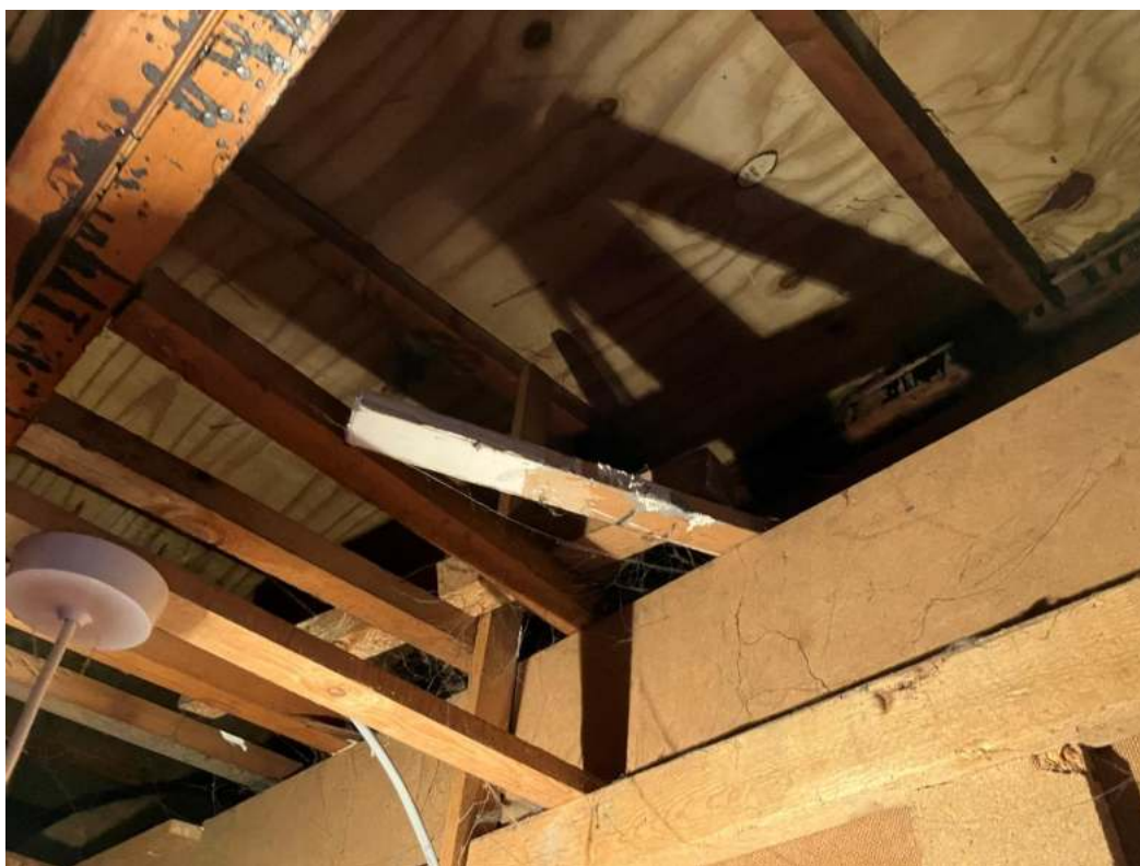
Internal view of flat roof over first floor to rear of two storey retail units
