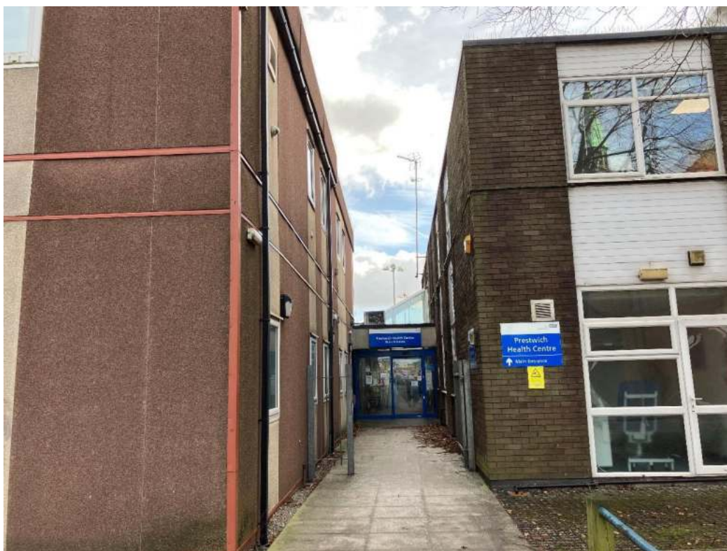
Main entrance to health centre from the north
