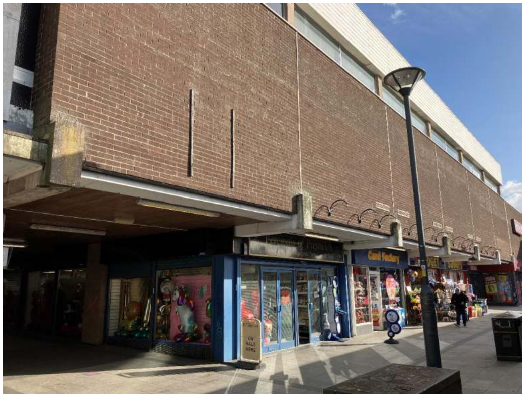
External western elevation of main event hall above ground floor retail units
