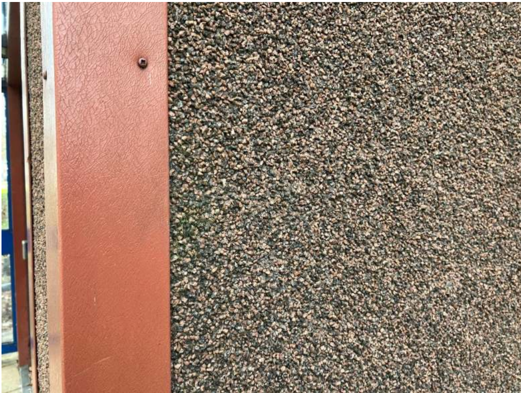
External cladding detail
