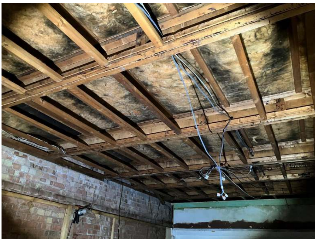
Internal view of flat roof after ceiling and wall finishes stripped out - 1
