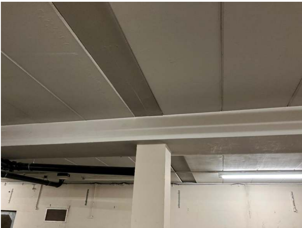
Roof planks supported on downstand beams with perpendicular tying beam at column location
