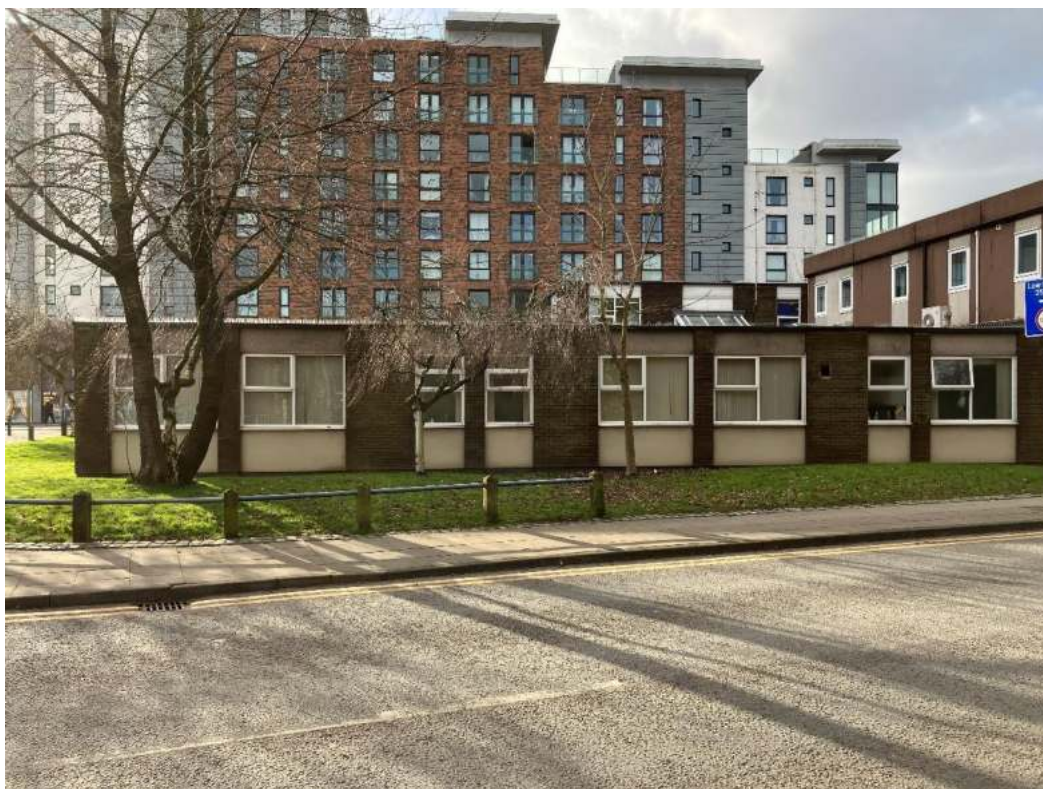
South east elevation of original single storey part of health centre
