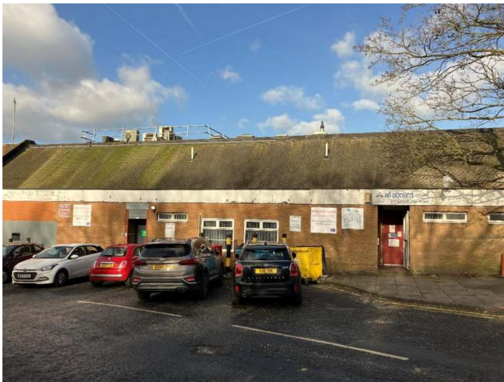
Rear elevation of double storey retail units 1
