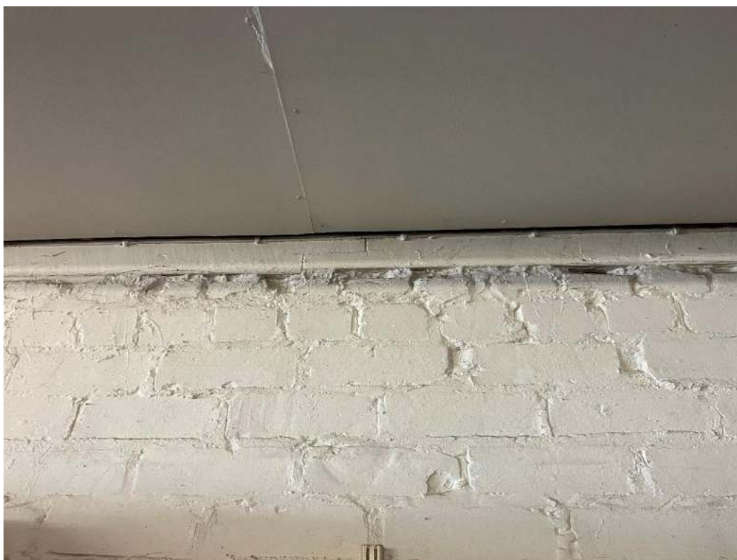
Head detail of party wall between adjacent retail units
