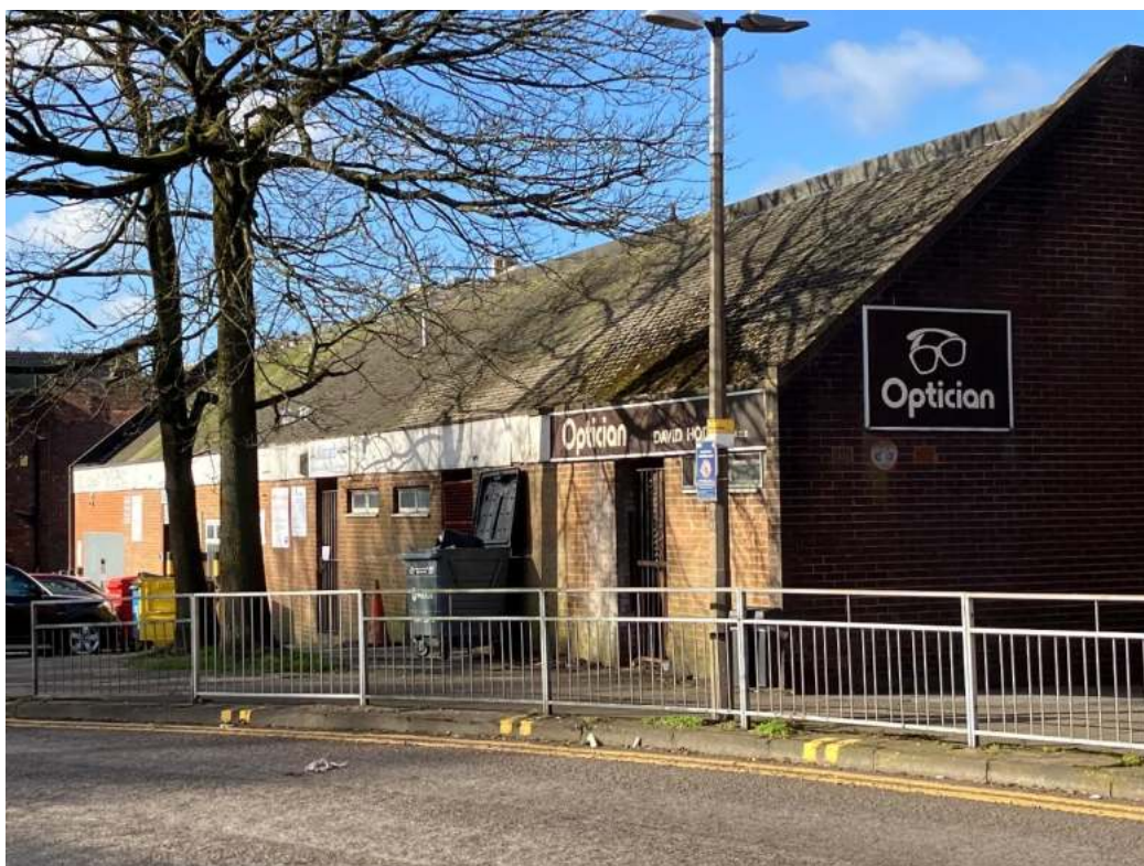
Rear elevation of double storey retail units 1
