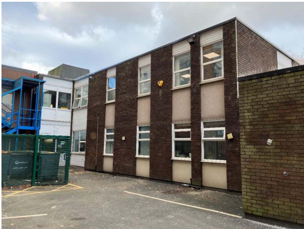
Original two storey section of health centre
