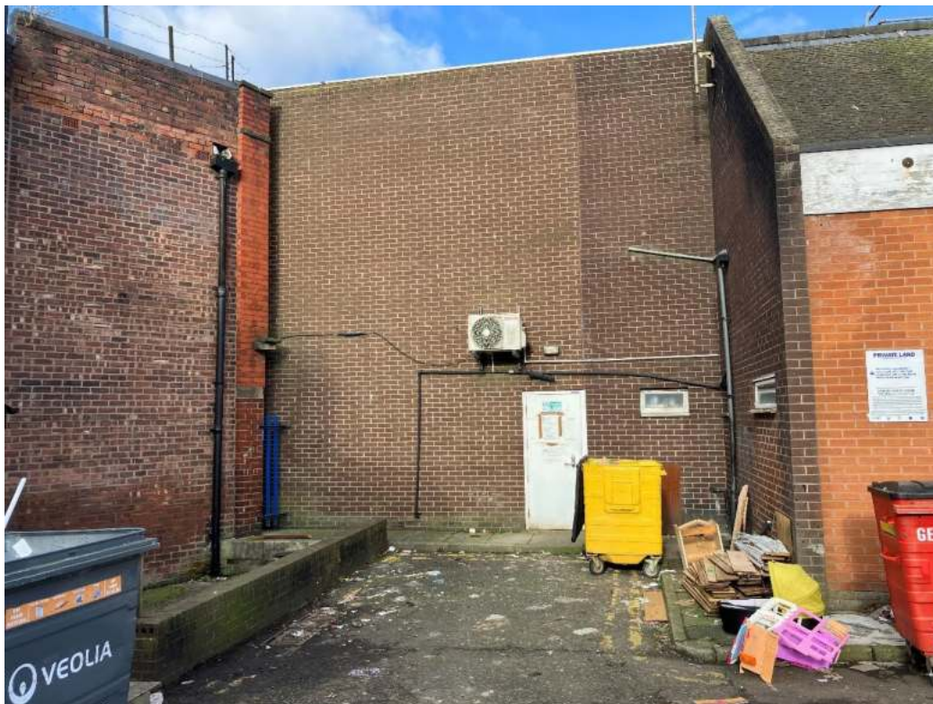
South (rear) wall to west end of double storey retail units
