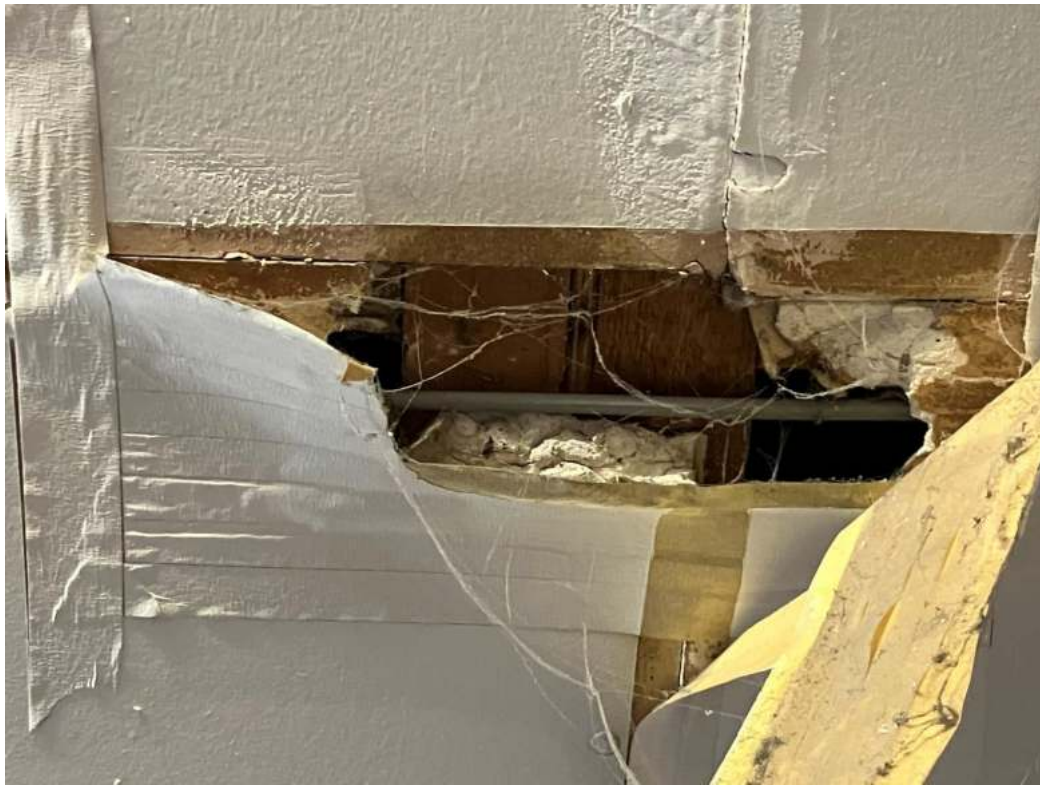
Locally opened up ceiling exposing composite timber "I" beam to roof
