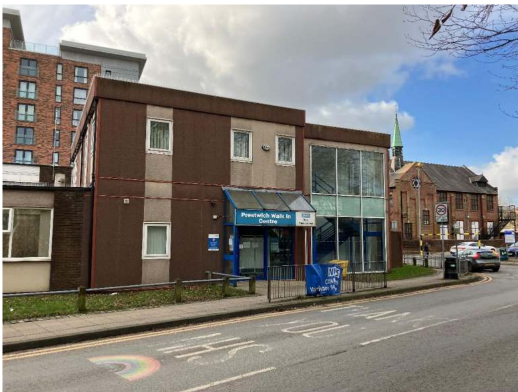
Eastern elevation of modular extension to north east of health centre
