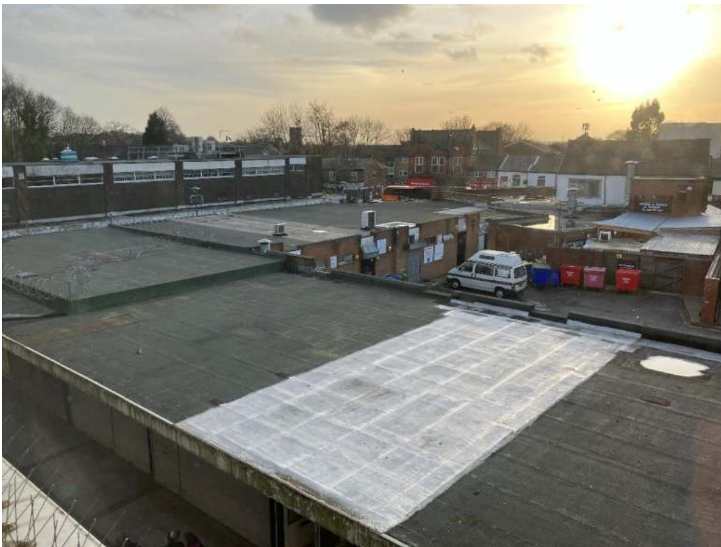
Flat roof to southern single storey retail units
