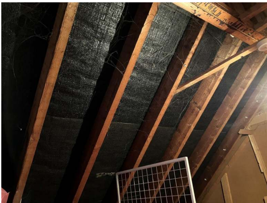
Internal view of sloping roof to rear of two storey retail units
