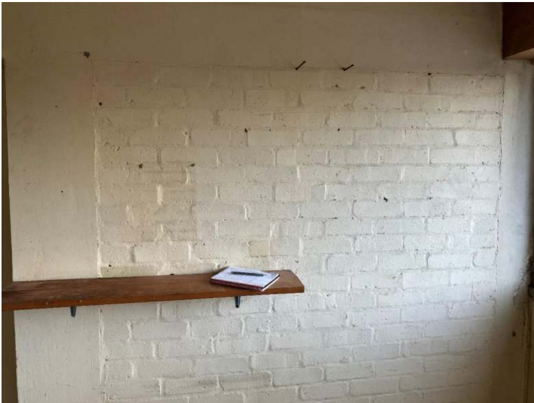
Internal second floor masonry infill wall within concrete frame
