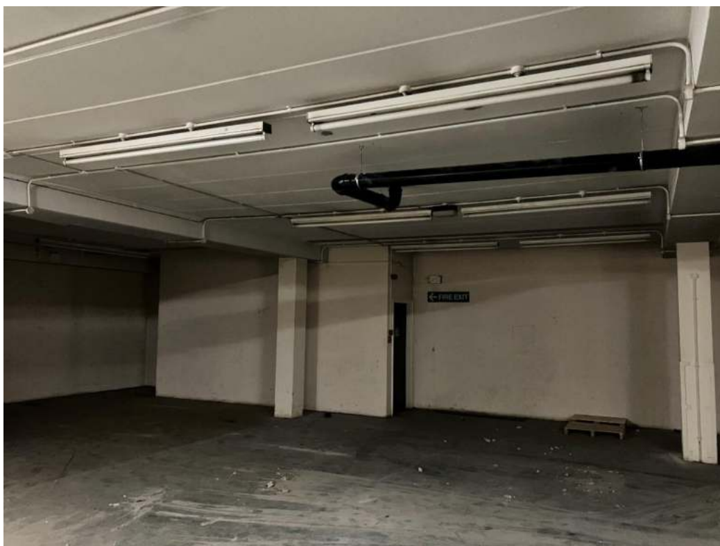
General view of first floor with exposed roof structure
