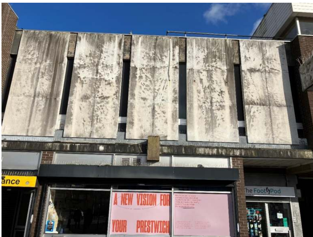
Precast concrete panels to first floor west elevation above ground floor retail units
