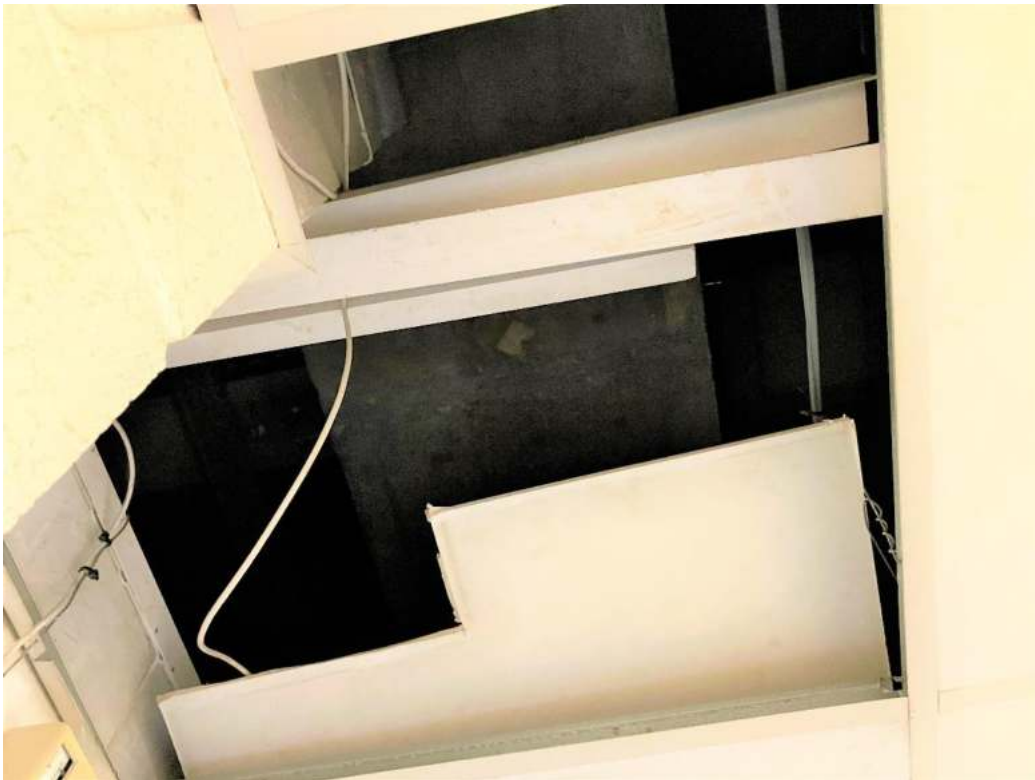
Downstand beam to first floor soffit revealed through locally opened up ground floor ceiling
