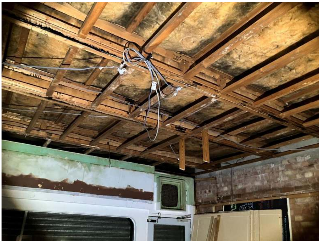
Internal view of flat roof after ceiling and wall finishes stripped out – 2
