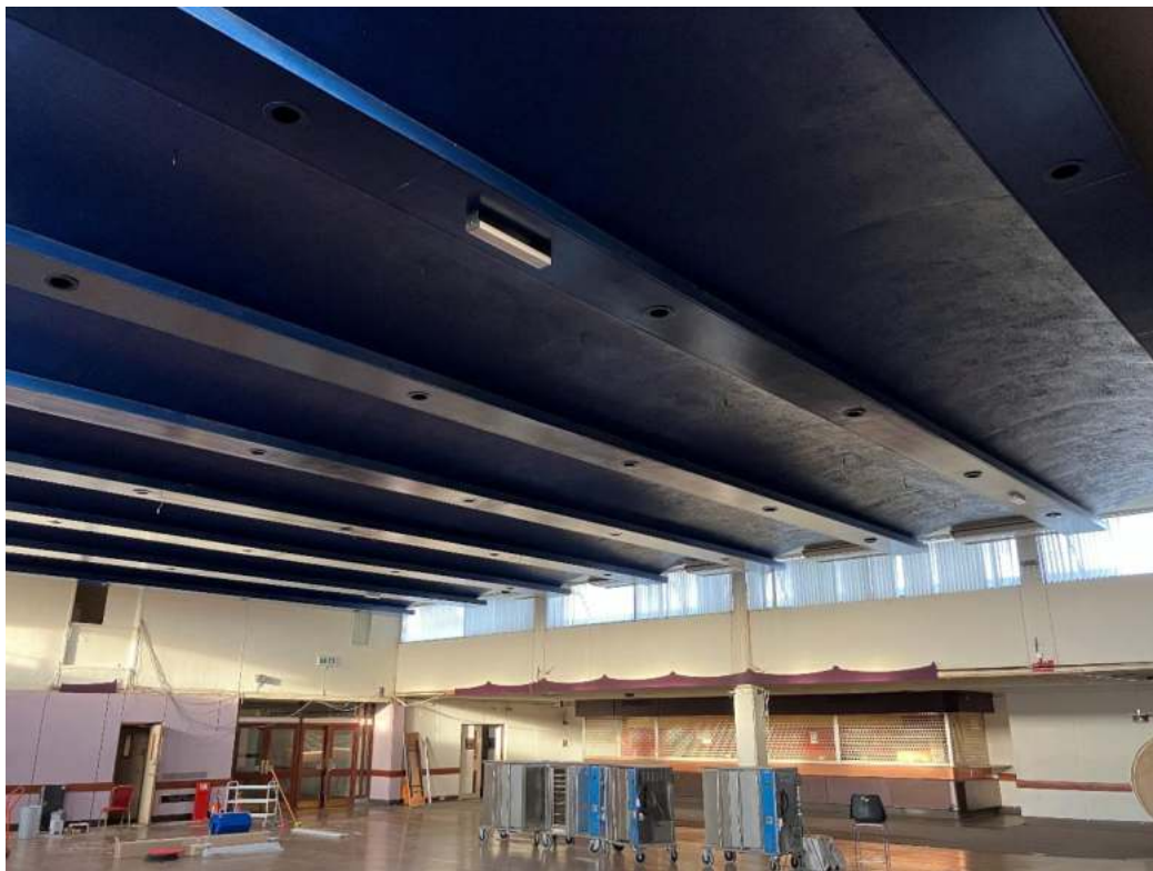
North-east view of main event hall
