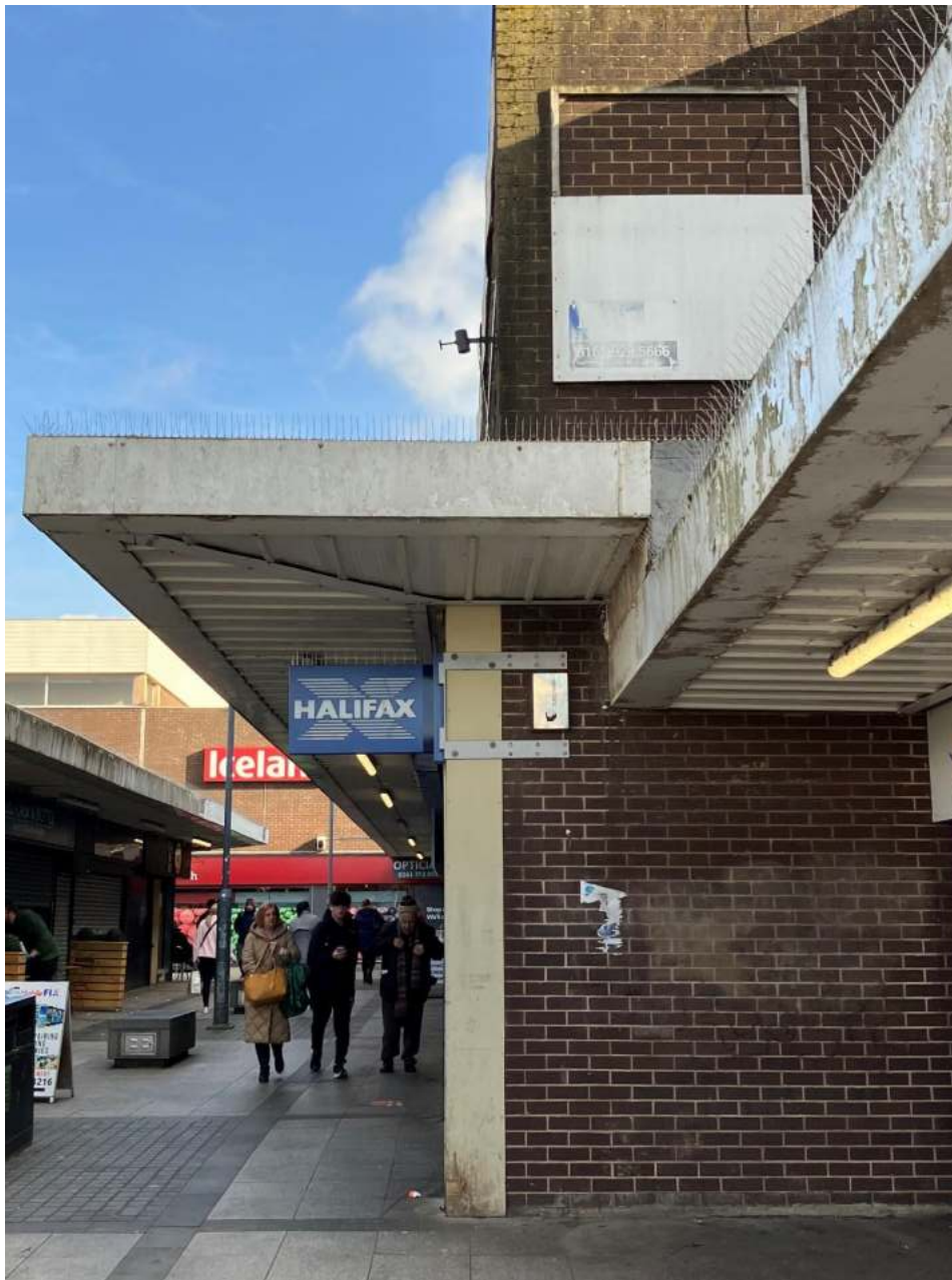
Cantilever canopy to double storey retail units
