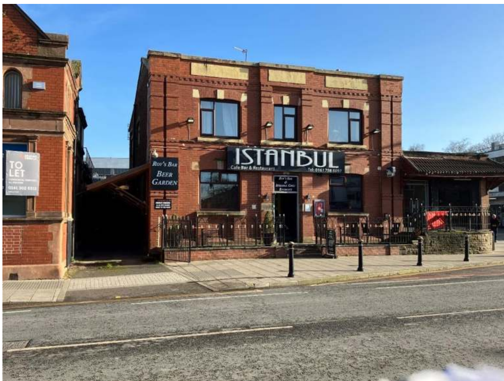
Front elevation of “Istanbul” restaurant
