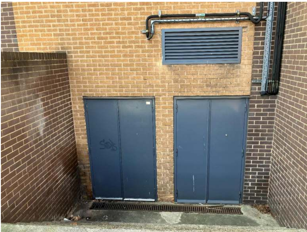
Fire escape doors into external recessed area in south east corner of store
