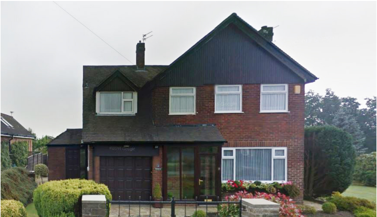
Existing view along Windrush Avenue
