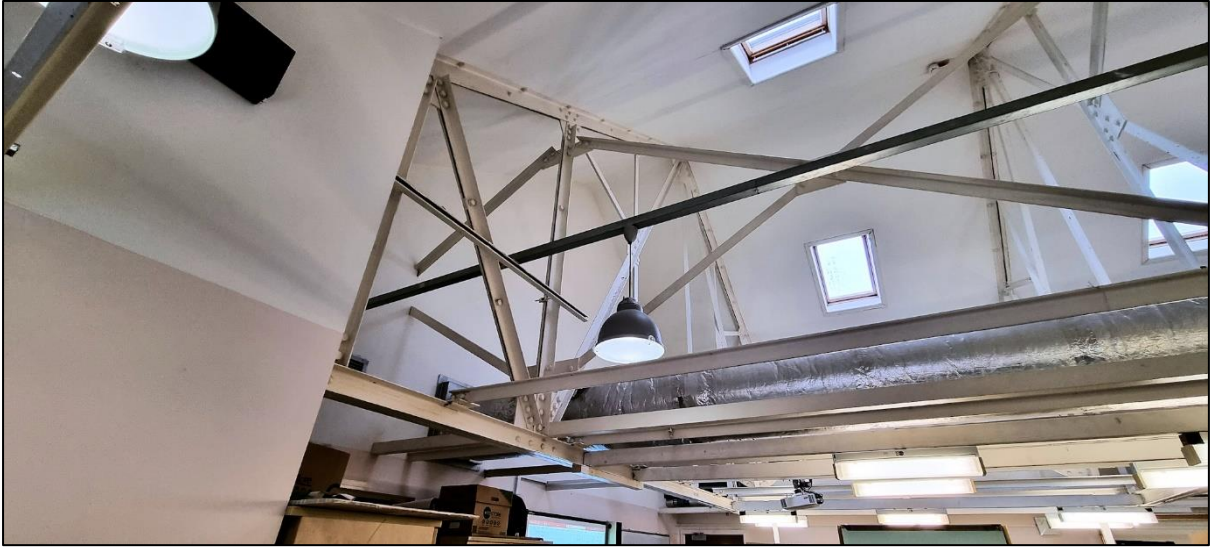
Plate 20: The upper floors had vaulted ceilings with no access to the underside of the roof.
