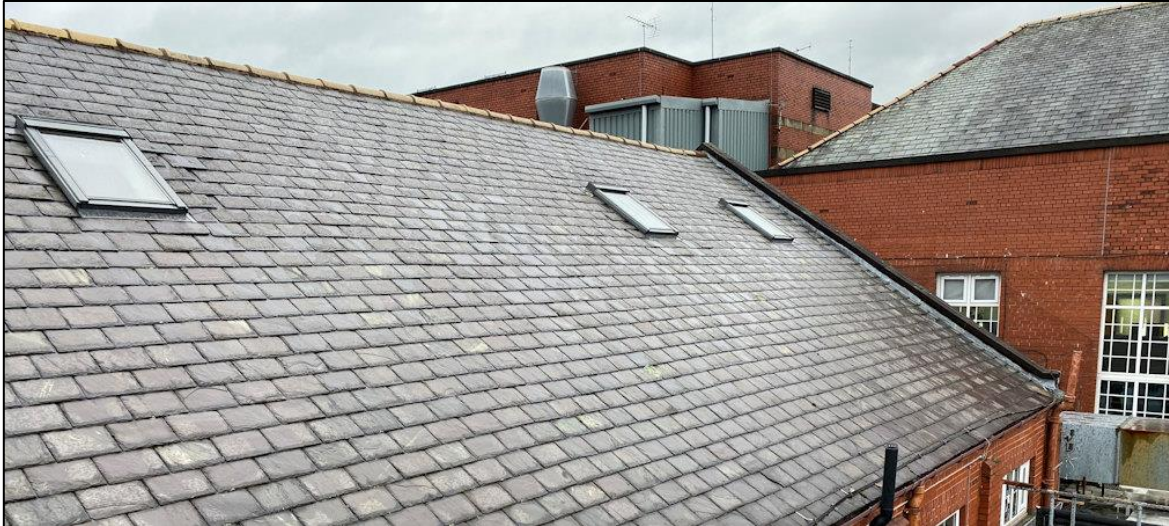
Plate 3: The pitched roof was generally intact.
