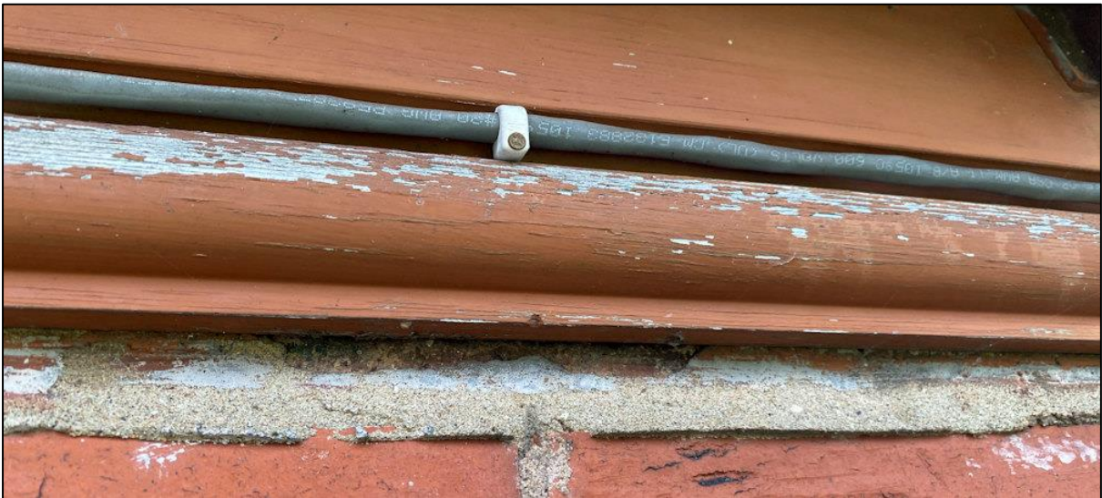
Plate 10: The fascia were intact with no PRFs and no roosting opportunities.
