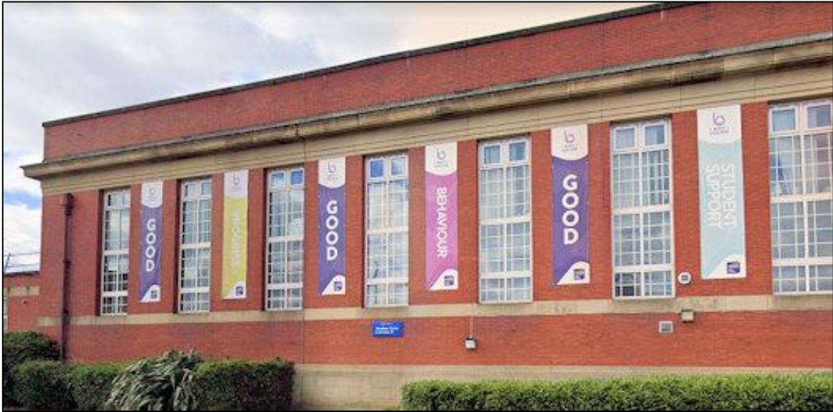
Plate 15: Windows to the front aspect of the complex were also well sealed and had no bat roosting potential.
