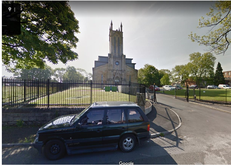
Image 1 – St Paul Court (formerly Church) – The Heritage Asset
