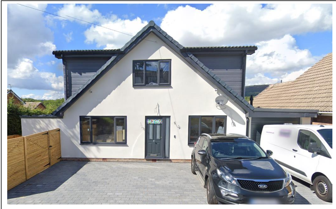
Figure 6. No. 1 Hargate Close
