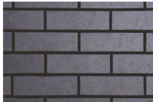
Brickwork - Staffordshire Blue Engineering Brick
