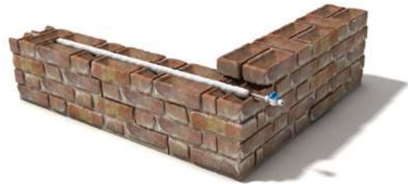
Stitching a cracked solid wall.
