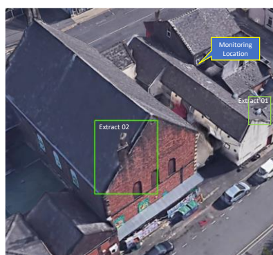
Figure 5 Rear of former church showing existing chimneys
